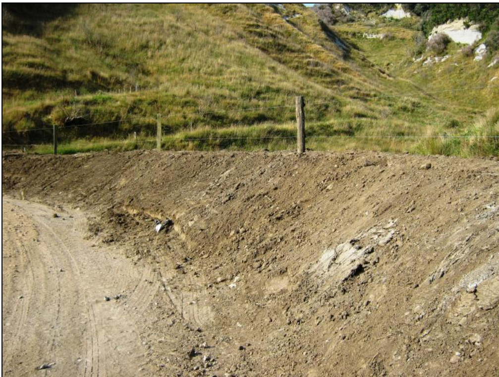
Photo 3 New retention bunding on track around pad one
