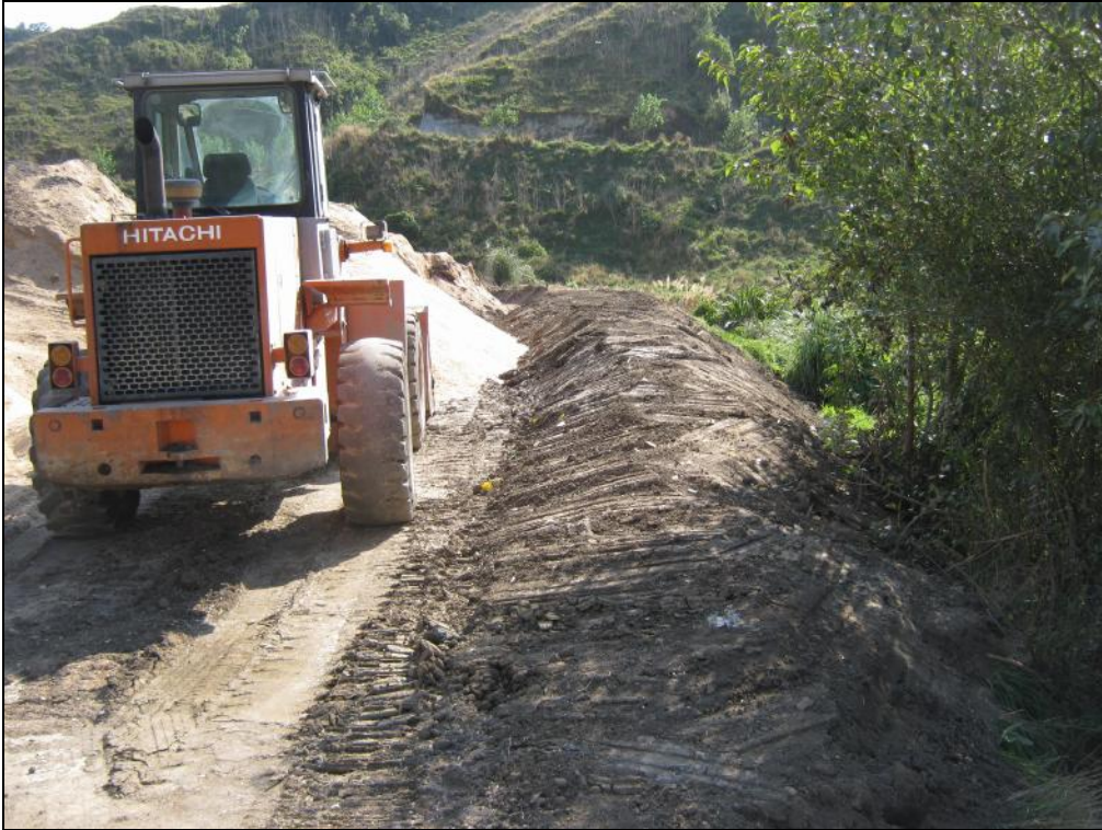
Photo 2 New retention bund along stream bank next to drilling waste pad
