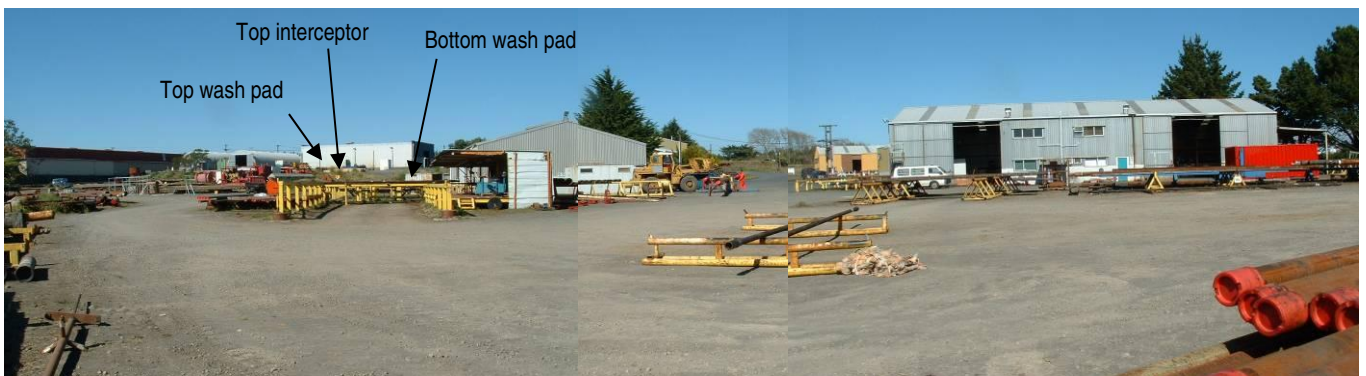
Photo 8 Weatherford New Zealand Ltd site - view from the northern corner
