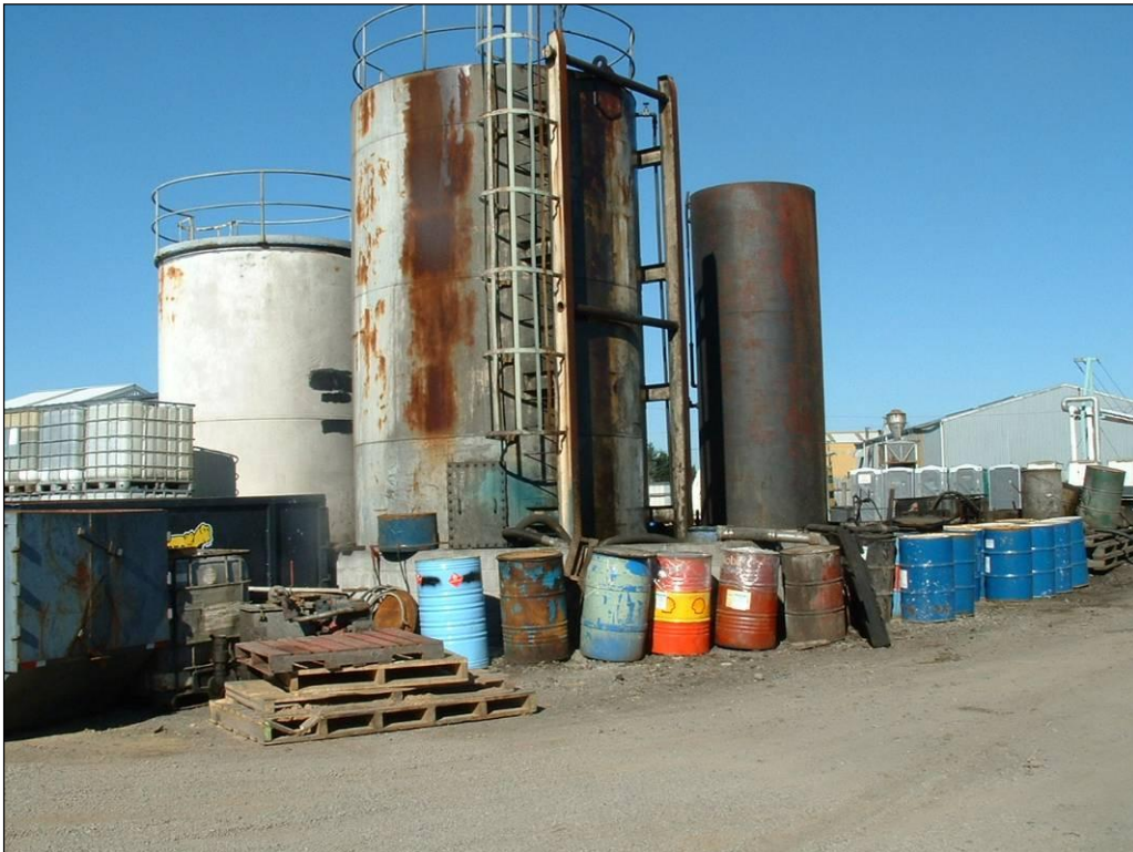
Photo 6 Transpacific Industrial Solutions waste oil storage
