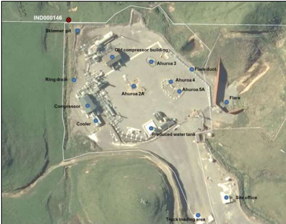
Figure 3 Ahuroa B wellsite and gas storage facilities showing main components and discharge sampling site IND000146
