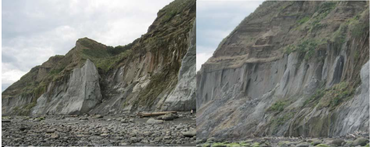
Photograph 8 Erosion of the cliffs close to 350m NW site (2013)
