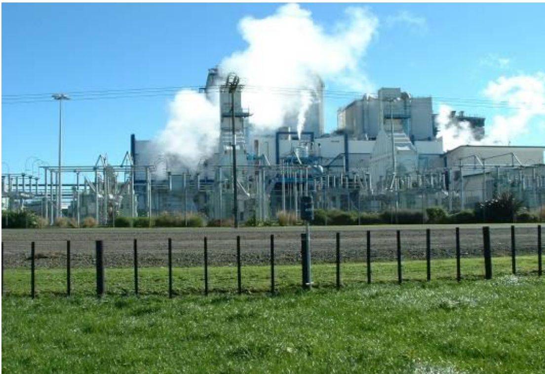
Photograph 3 Air discharges from 'Cogen-I' and 'Cogen-II'
