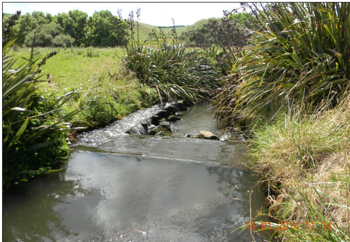
Photo 1 The weir and fish pass on the Tawhiti Stream
