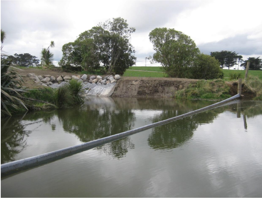
Photograph 6 Tawhiti stormwater pond following remedial work
