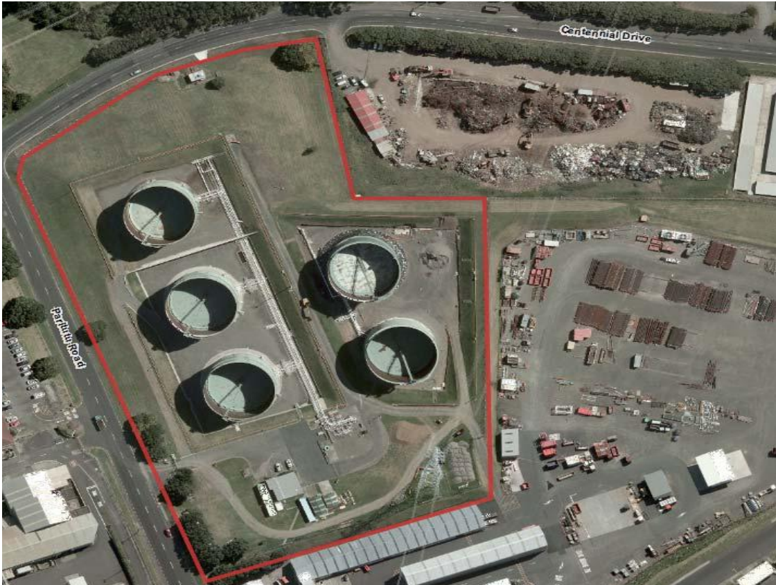
Figure 7 Aerial photograph of the Shell Todd Oil Services Ltd Paritutu Tank Farm
