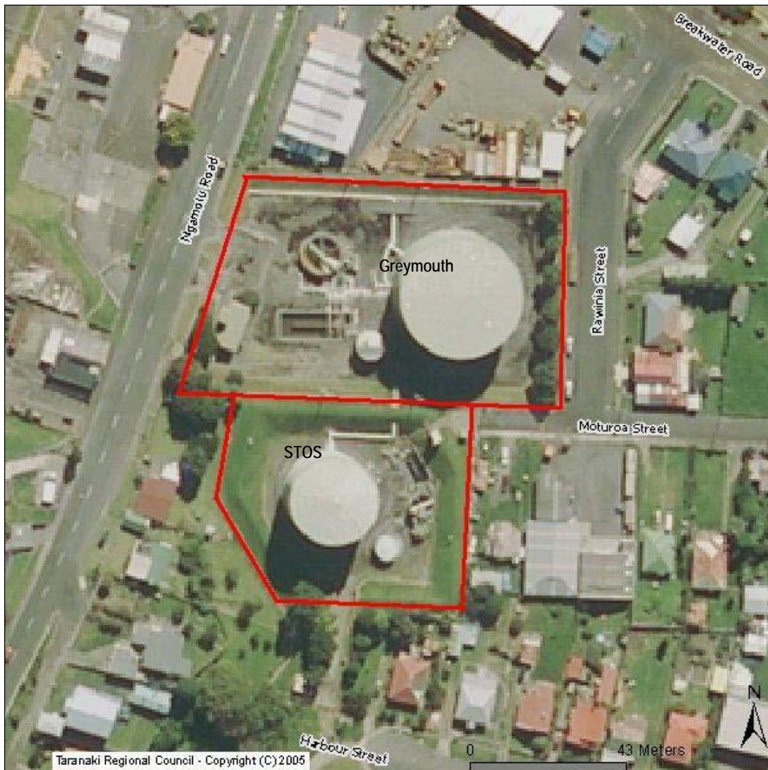
Figure 5 Aerial photograph of the Greymouth and STOS deballast sites
