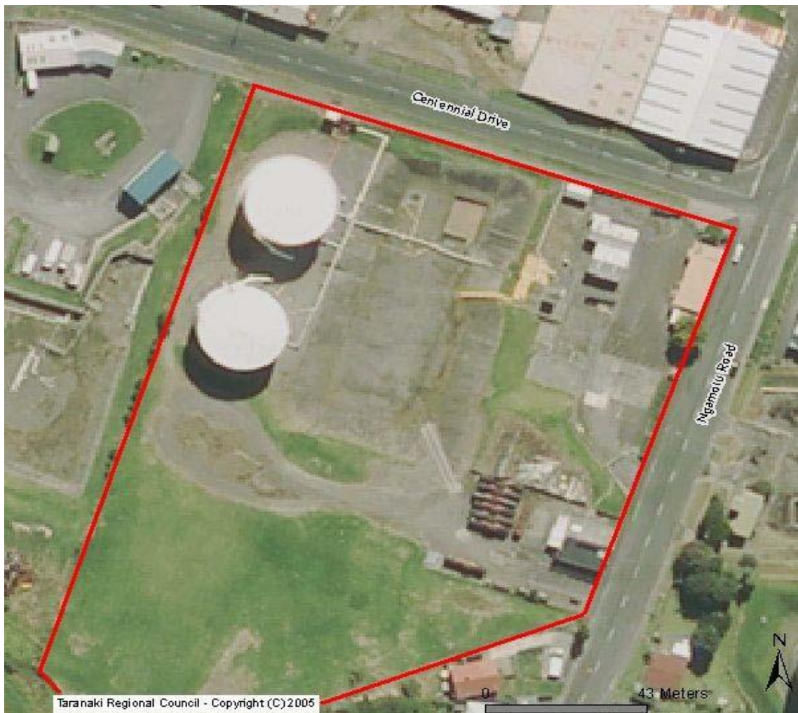
Figure 6 Aerial photograph of the New Zealand Oil Services Ltd Ngamotu Road site
