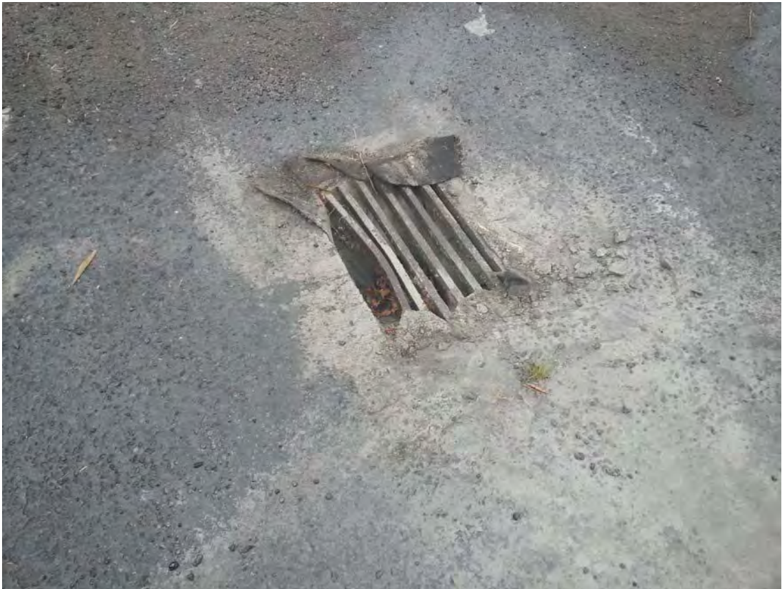
Photo 5 Halliburton stormwater drain 18 March 2014
