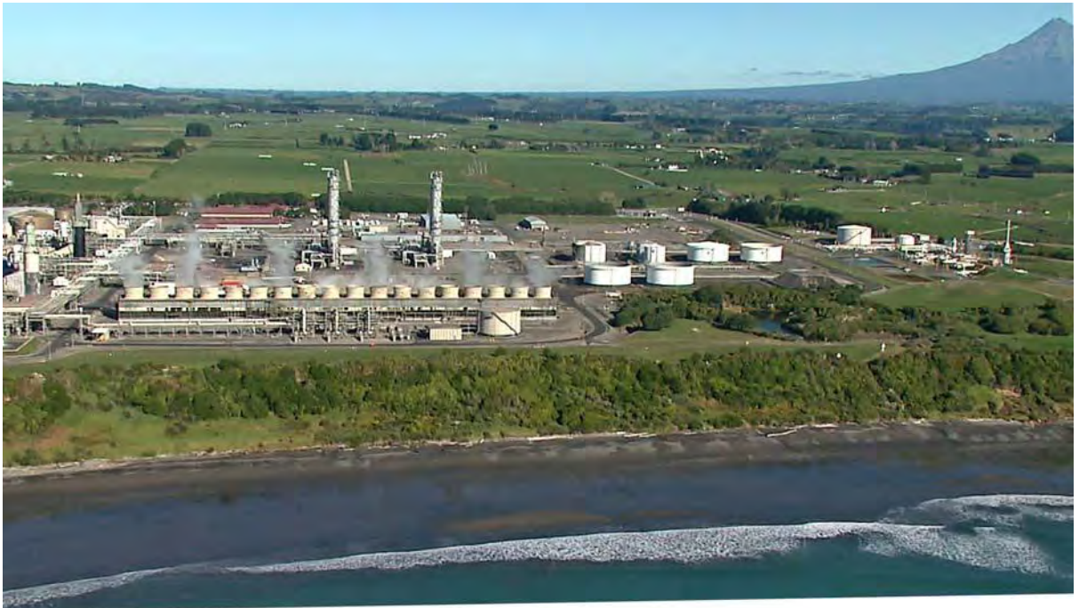
Photo 1 Cooling towers and distillation stacks at the Methanex Motunui plant
