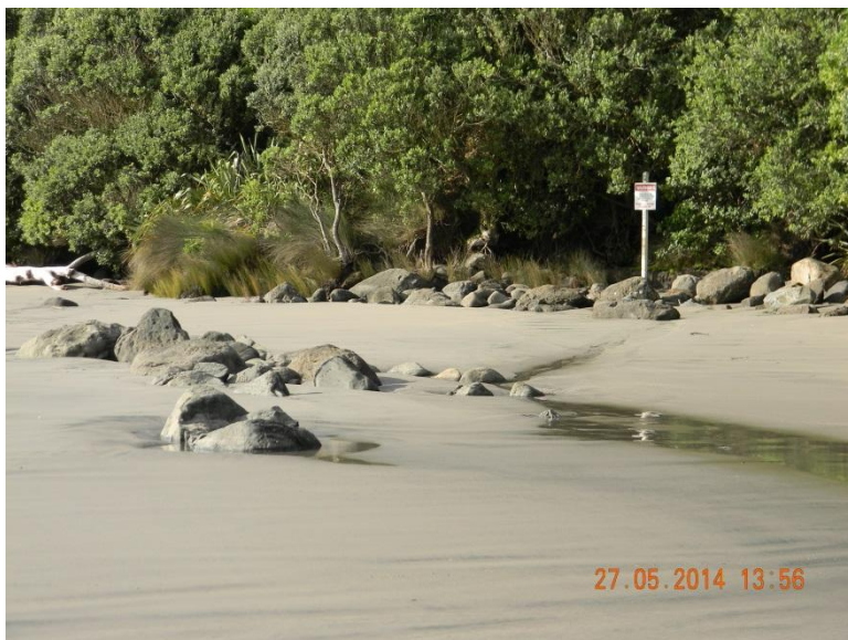
Photo 6 The location of the station outlet on Opunake Beach completely buried in sand. Note the warning sign in the background, erected in compliance with consent 4744-4
