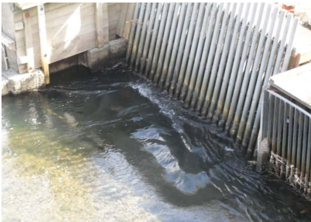
Photo 2 The river intake during high lake levels (top left) and low lake levels (right). The intake tunnels that carry water to the canal are located immediately behind the intake screen.
