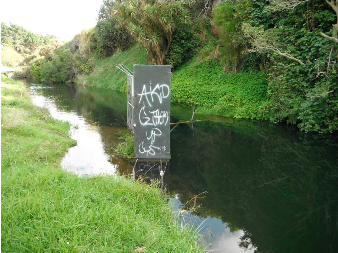
Photo 7 The intake canal on 23 April 2012 looking towards Opunake Lake.
