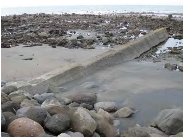
Photograph 5 Sand accumulation observed on the high-shore at Arakaitai in 2010
