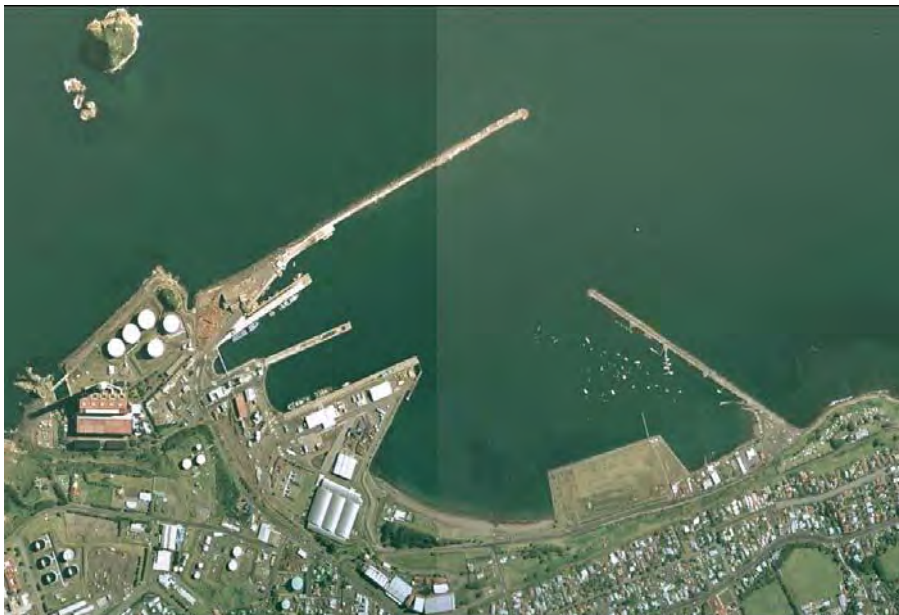
Figure 1 Port Taranaki showing the Main Breakwater on the left and the Lee Breakwater on the right
