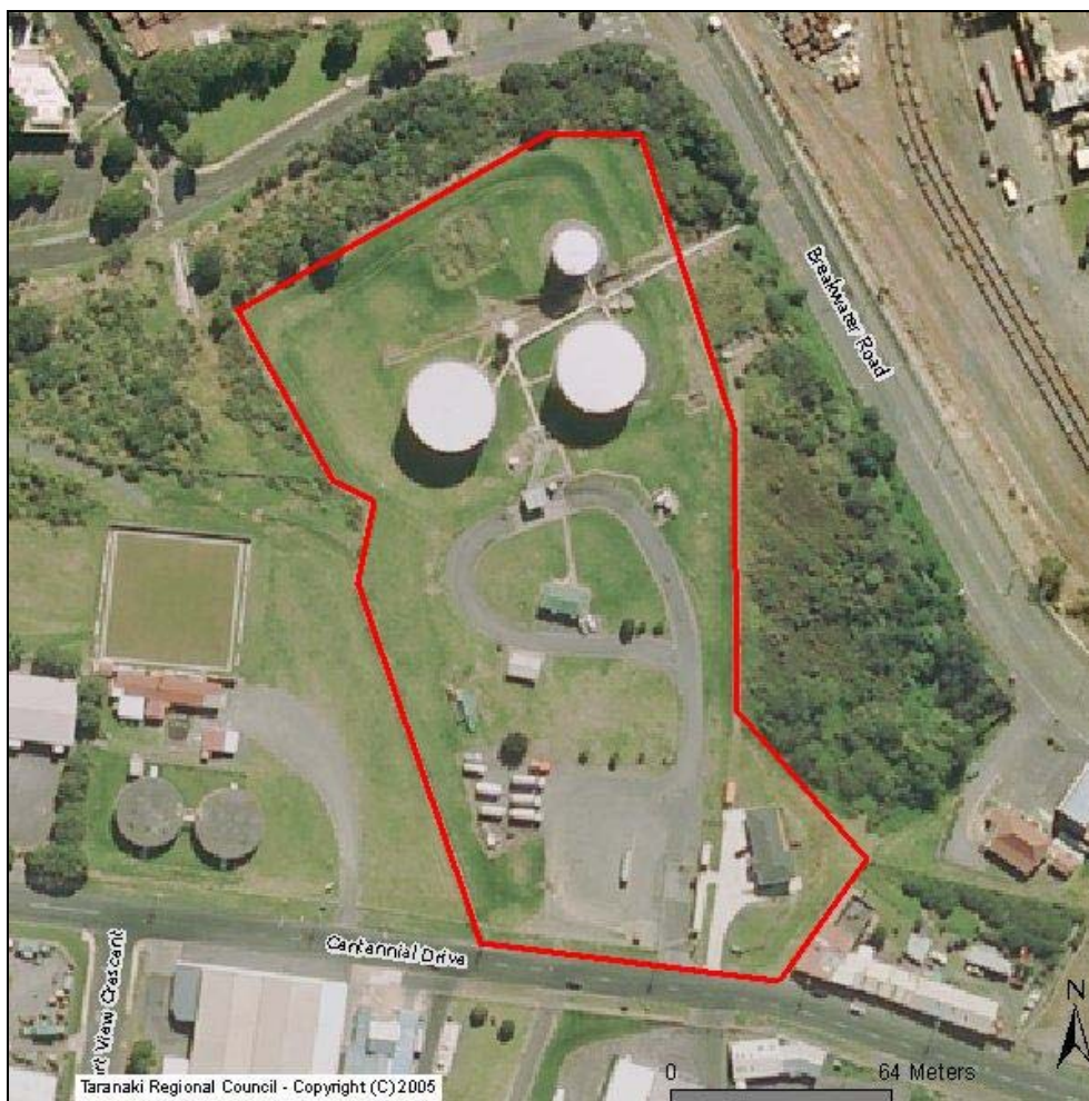
Figure 3 Aerial photograph of the New Zealand Oil Services Limited Centennial Drive site
