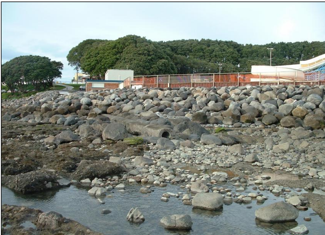
Photograph 1 Todd Energy Aquatic Centre ocean outfall
