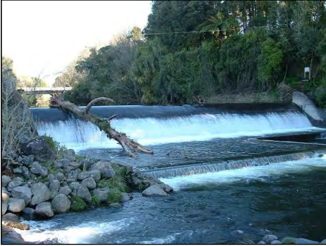
Photo 6 The Tariki Weir, 29 June 2012
