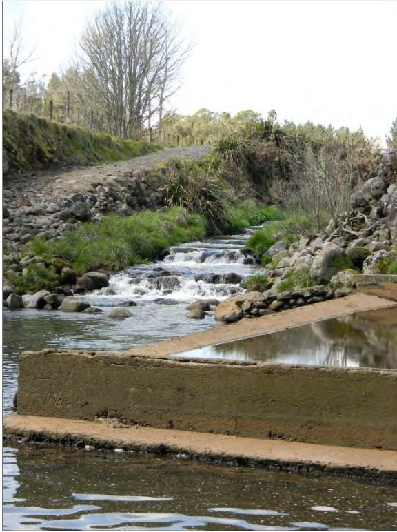
Photo 11 The outlet of the Tariki Weir fish pass
