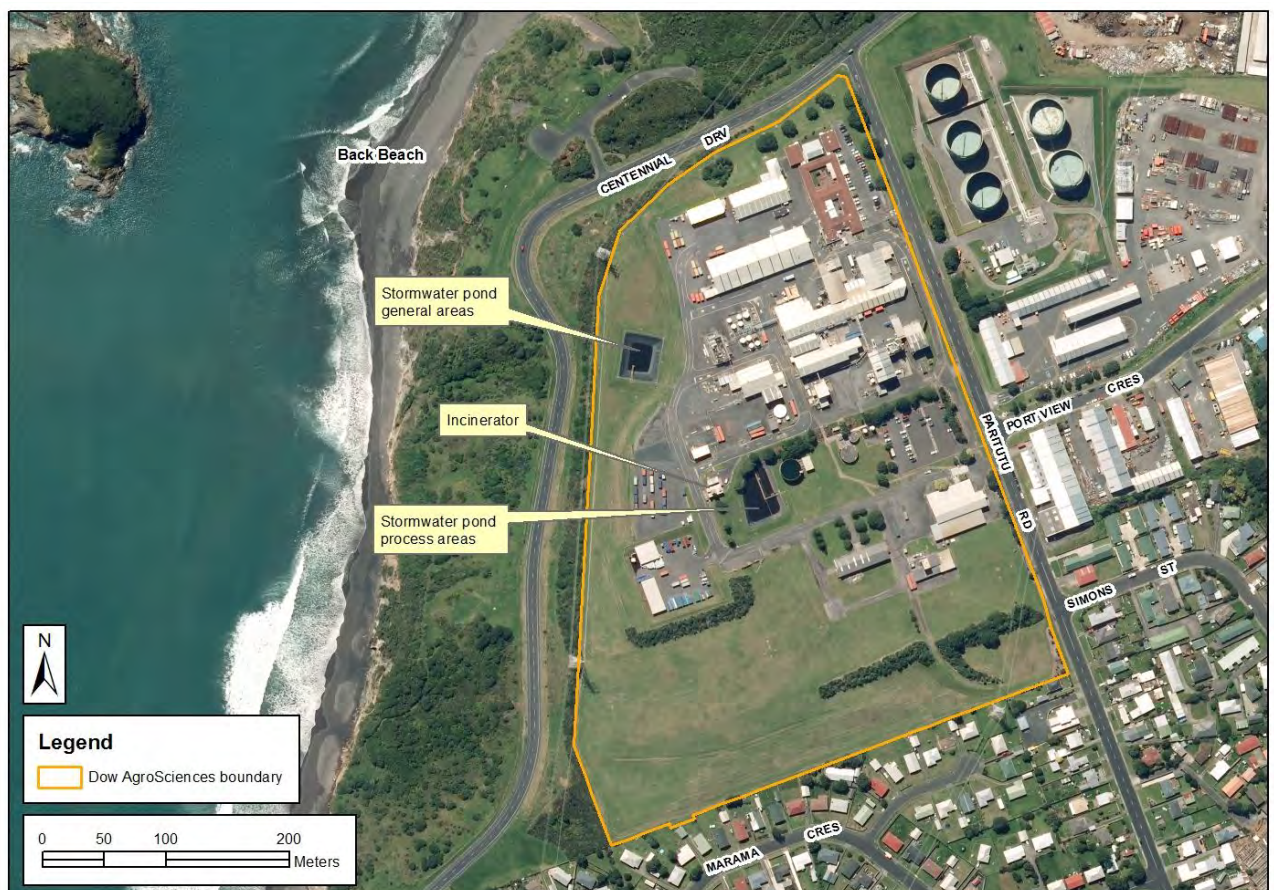
Figure 1 Aerial photograph of Dow AgroSciences site
