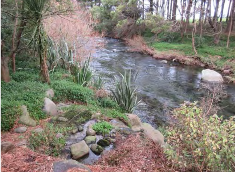
Photo 3 Outfall from stormwater pond to Kaipokonui Stream
