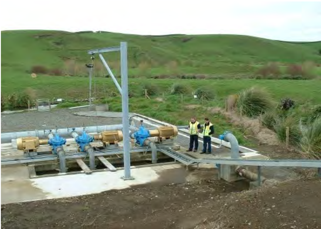
Photograph 2 Tawhiti water intake
