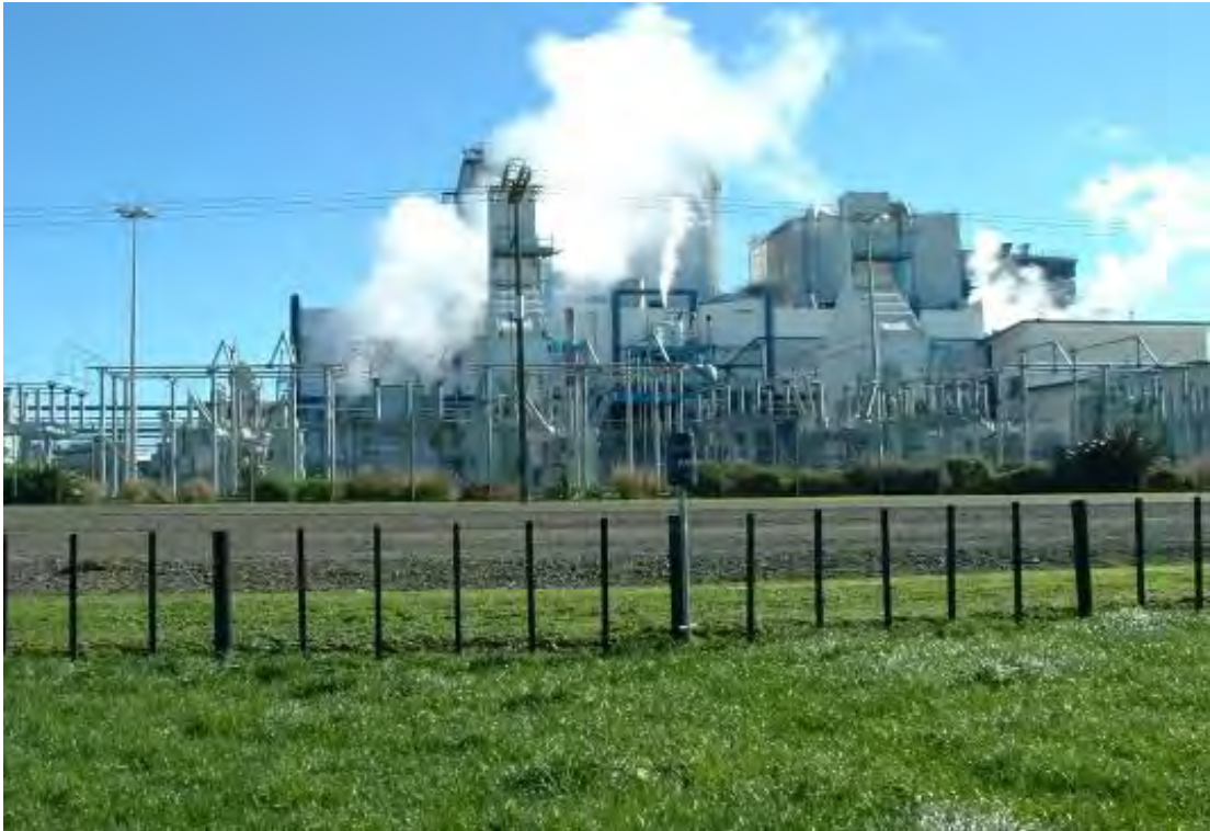
Photograph 3 Air discharges from 'Cogen-I' and 'Cogen-II'
