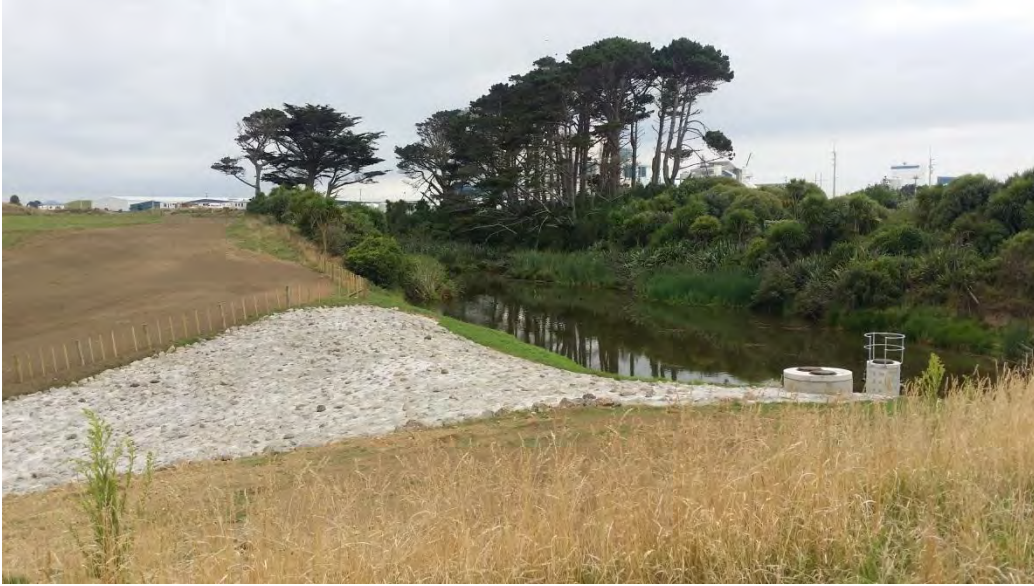
Photograph 6 Southern stormwater pond following upgrade (photo taken 12 March 2015)
