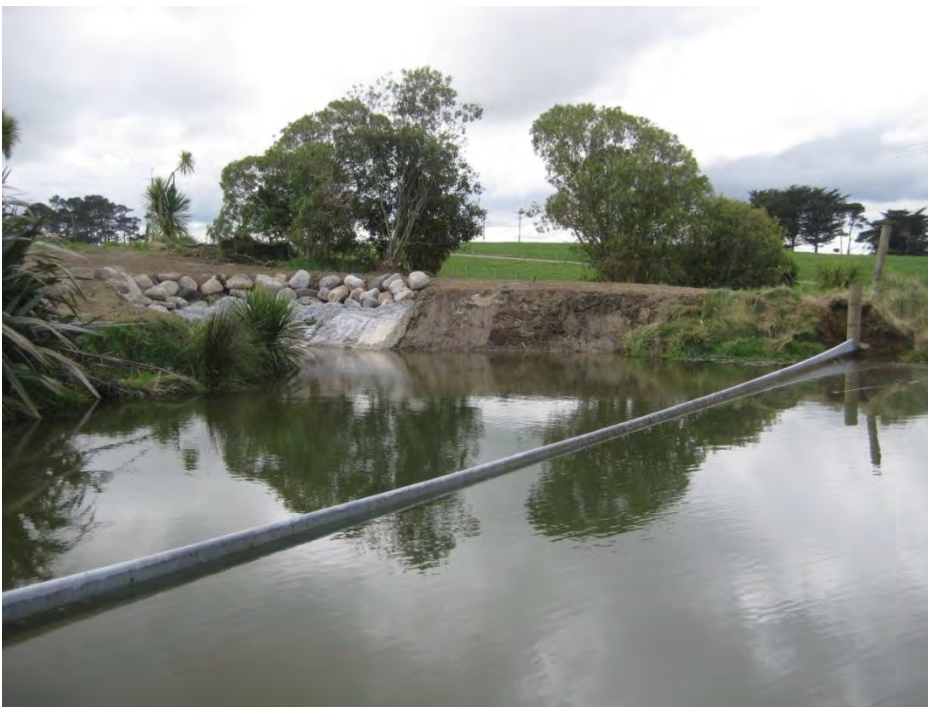
Photograph 7 Tawhiti stormwater pond following remedial work
