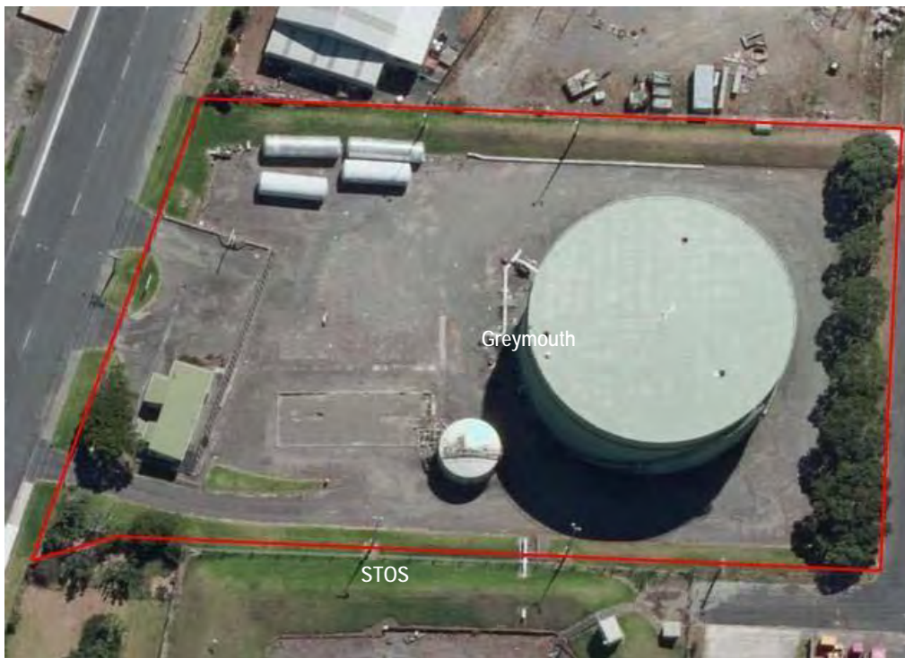
Figure 5 Aerial photograph of the Greymouth bulk storage facility
