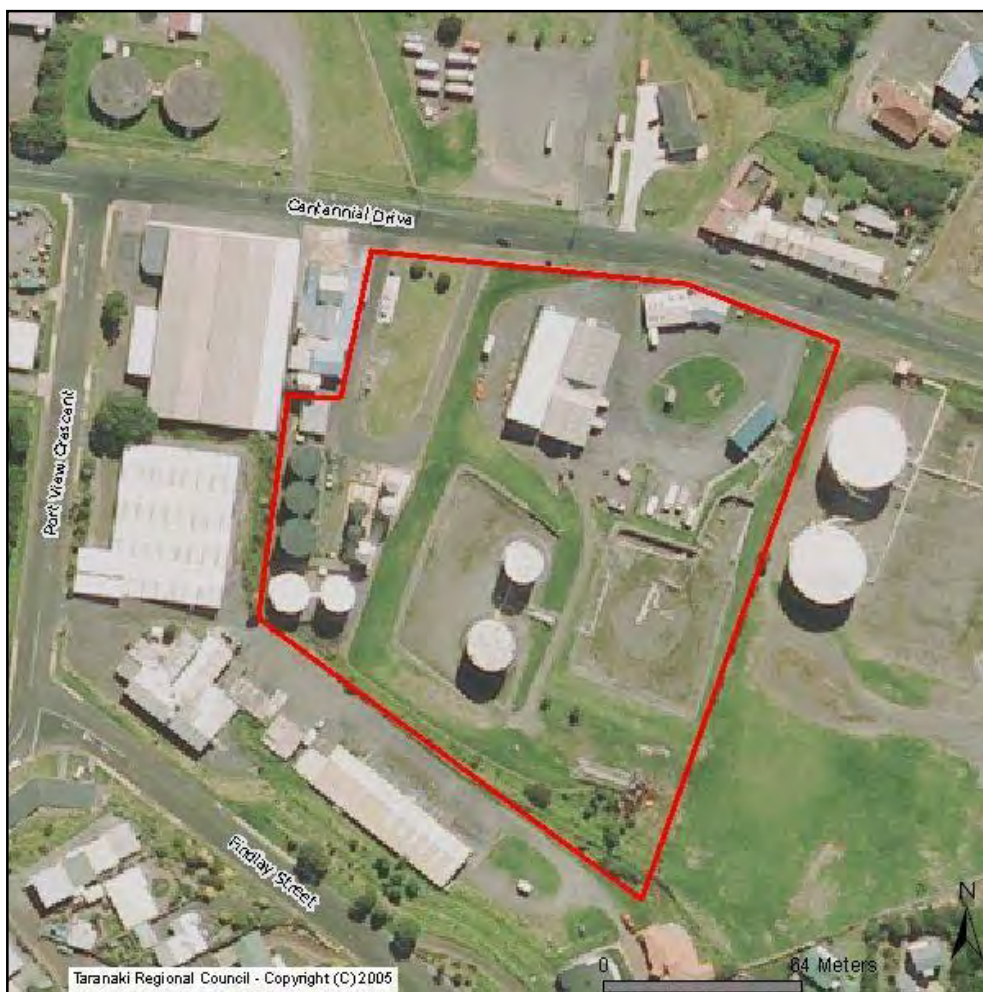
Figure 3 Aerial photograph of the Bulk Storage Terminals Ltd site
