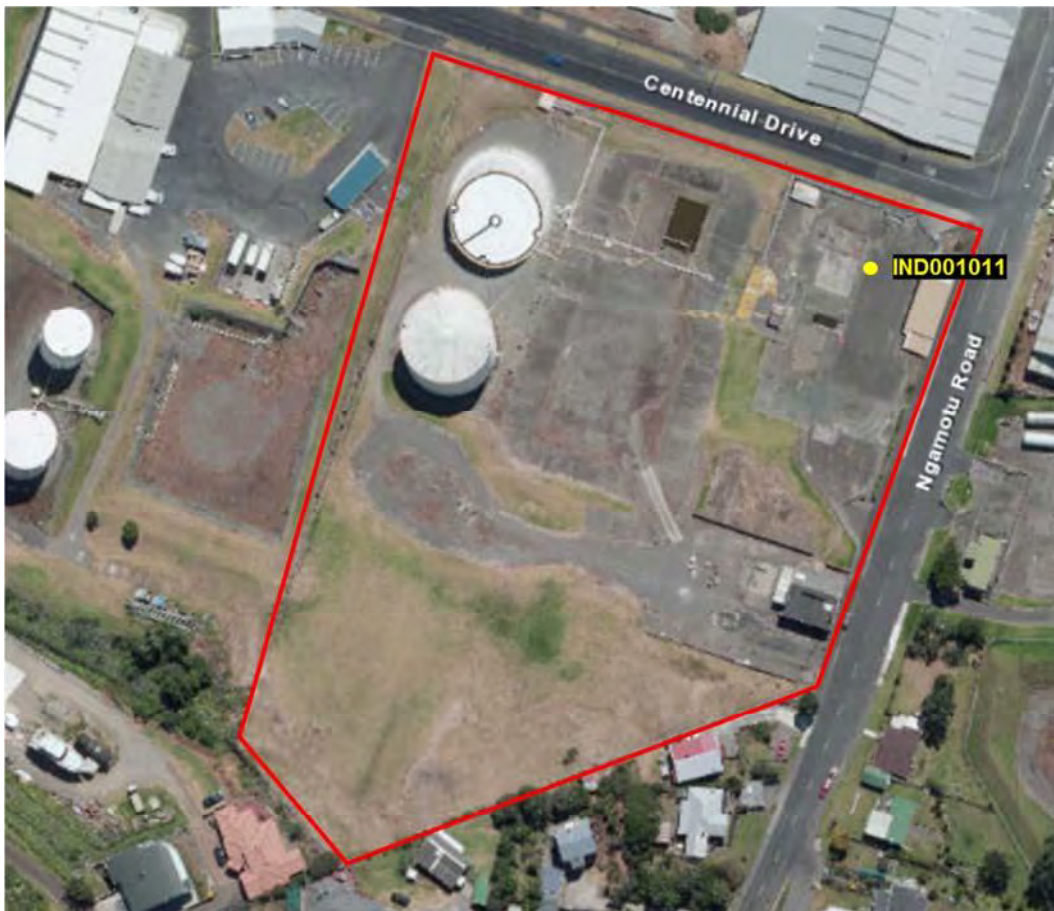
Figure 8 Aerial photograph of the New Zealand Oil Services Ltd Ngamotu Road site
