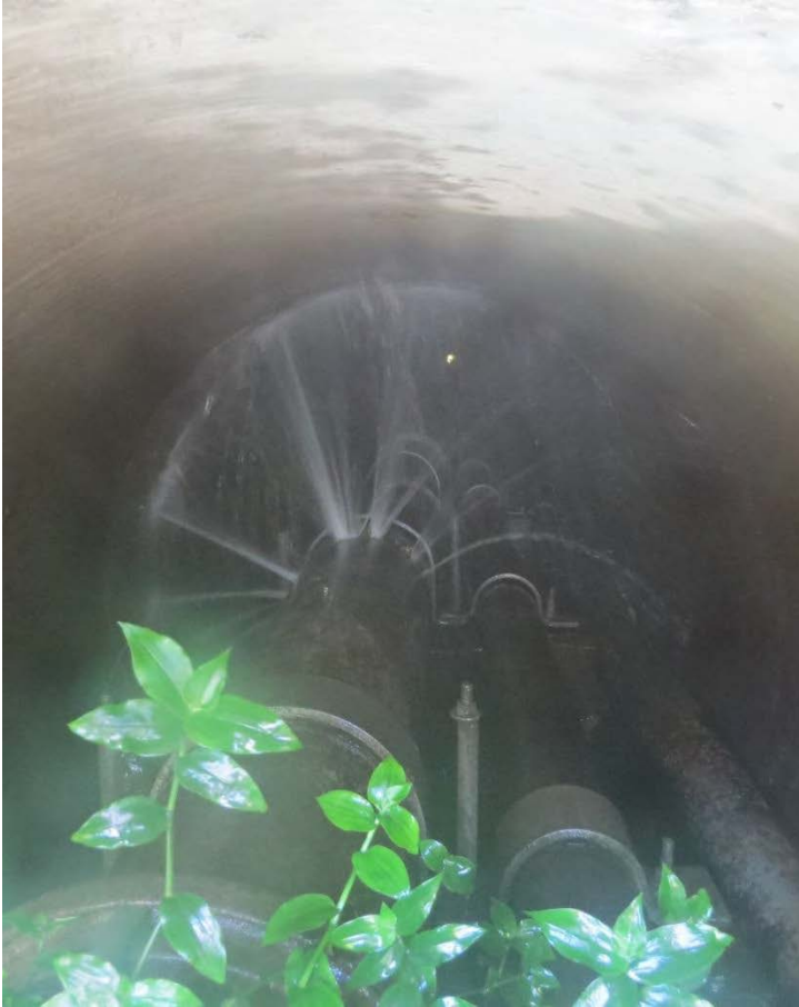
Photo 4 Point of discharge – Roadside culvert
