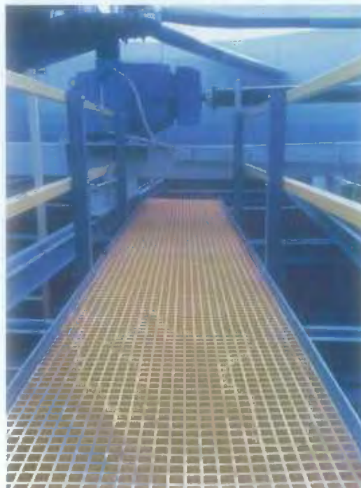
Picture1 – viewing from the fanstack access hatch
