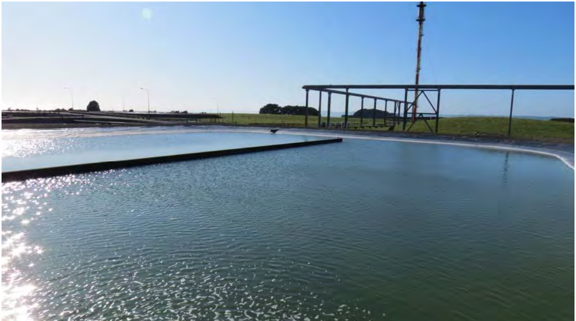
Photo 2 The Motunui plant's blow down pond (decommissioned flare 2 can be seen in the background)
