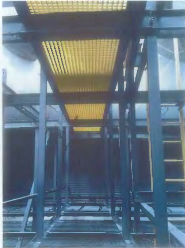
Picture 3 – viewing from below the access walkway Plenum above drift eliminators
