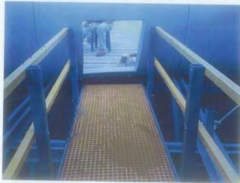
Picture 2 – viewing from inside the fanstack, from gearbox
