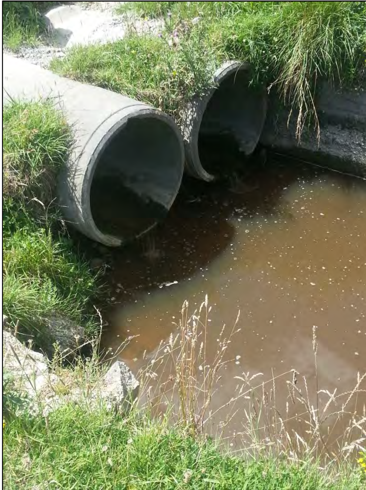
Photo 2 The access culvert immediately upstream of site 2.
