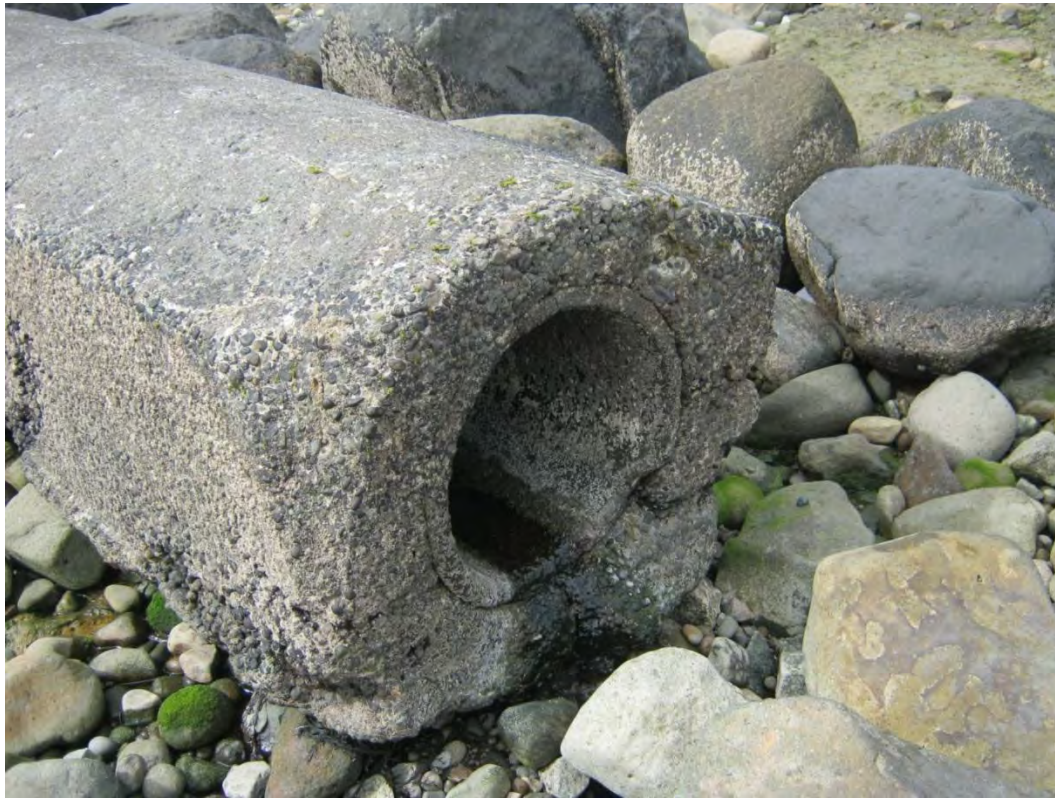
Photograph 2 Todd Energy Aquatic Centre discharge pipe
