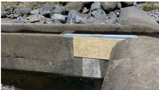
Photo 3 Repair to fish pass, early 2015
