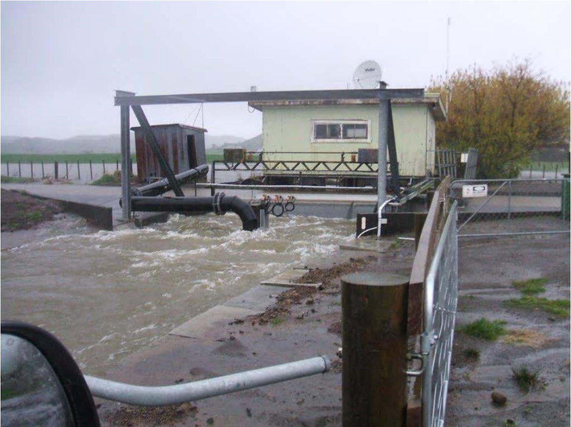
Photo 8 The Mangaotea Aqueduct, 20 June 2015.
