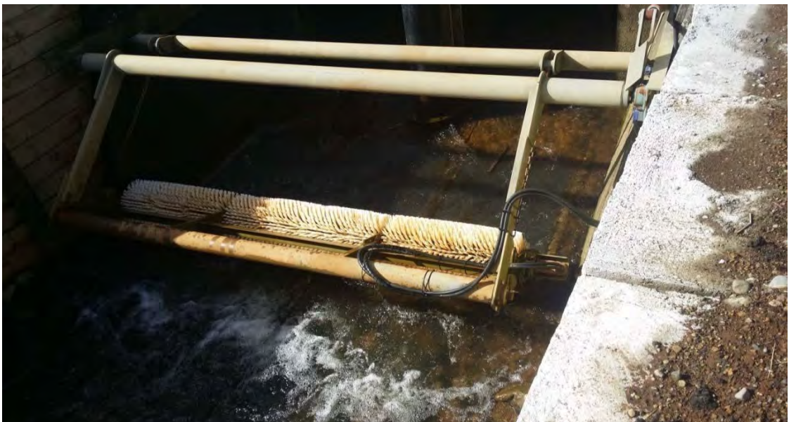
Photo 3 The Mangaotea Stream intake with the screen cleaner operating (below)
