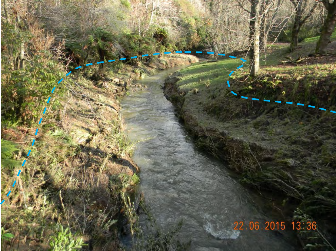
Photo 10 The Mako Stream bridge, Makara Rd, 22 June 2015. The blue line indicates the approximate flood height.
