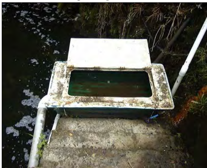
Photo 5 Elver trap at the base of the tail race at the power station
