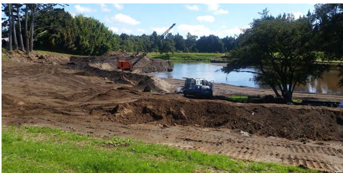
Photo 4 Dredging activities at Ayling's Pond.
