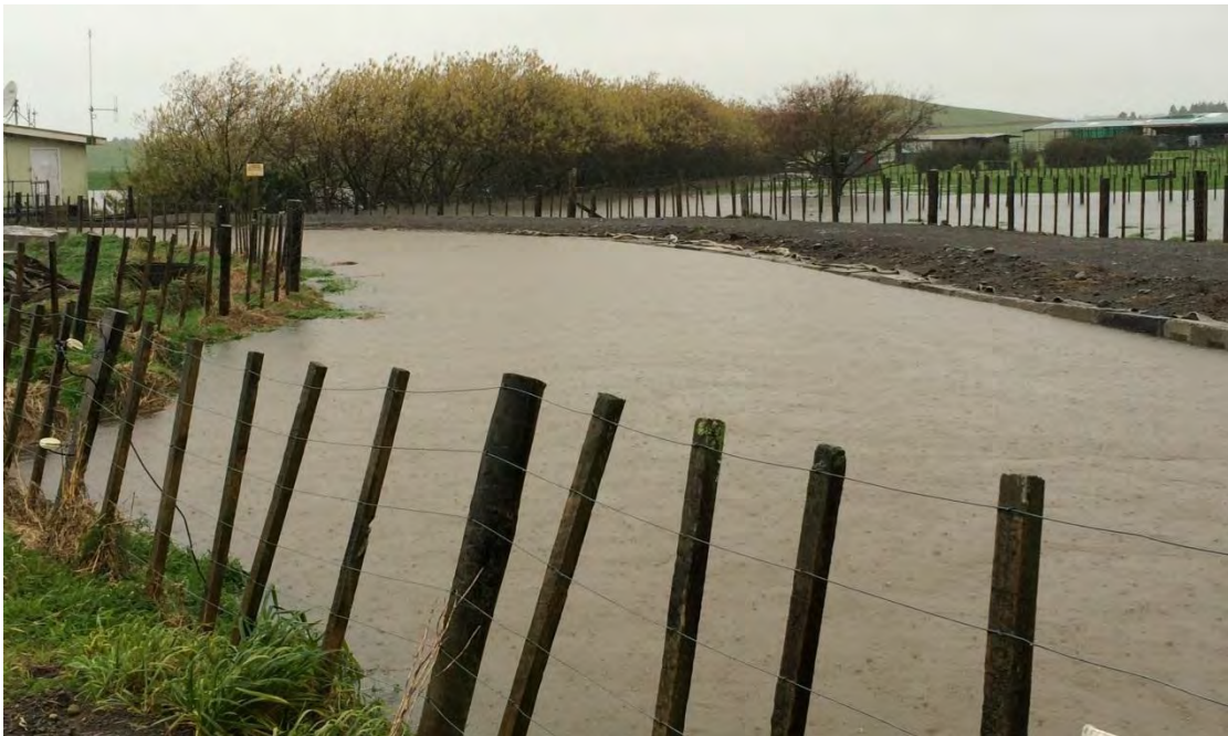
Photo 7 The Motukawa Race looking downstream from the Mangaotea Rd culvert, 20 June 2015.
