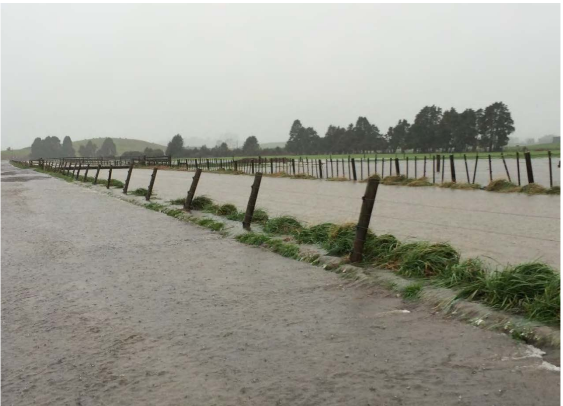
Photo 9 The Motukawa water race overflowing downstream of the Mangaotea Aqueduct, 20 June 2015.
