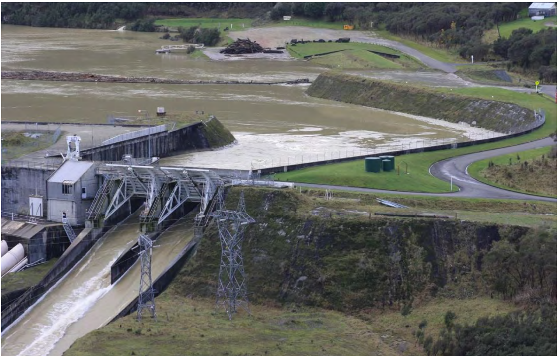
Photo 5 The Patea Dam spillway gates during the June 2015 flood event 4 . Note the spillway gates are open to the point of not restricting flow.
