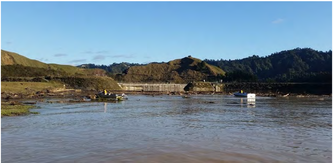
Photo 9 Boats clearing the logs at the Patea Dam log boom, 25 June 2015.
