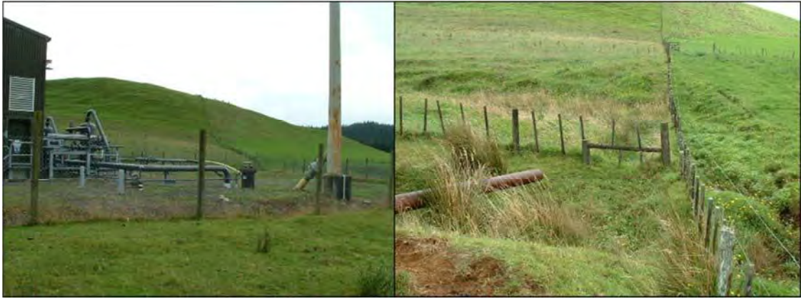
Photo 4 Ahuroa-B site looking towards skimmer pond (left) and final pond discharge point (right)
