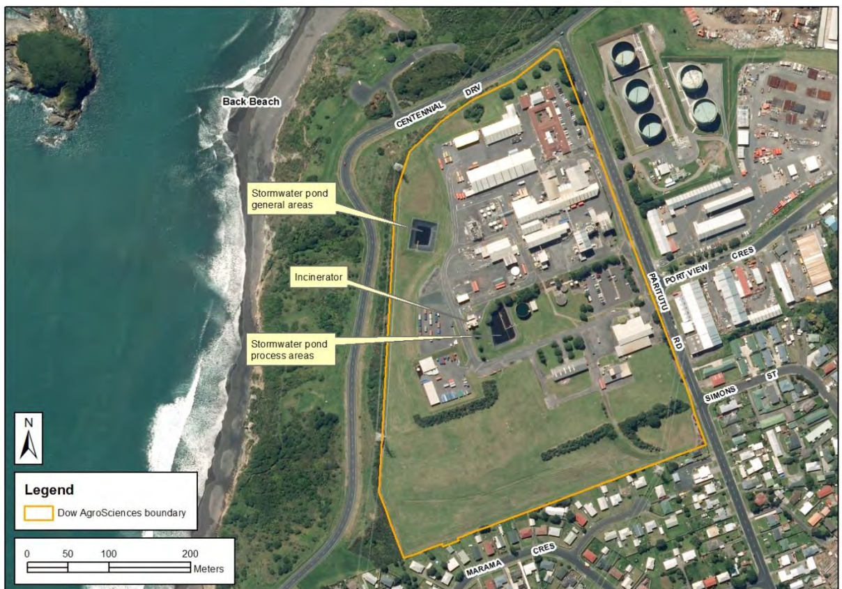
Figure 1 Aerial photograph of the DAS Paritutu Road site
