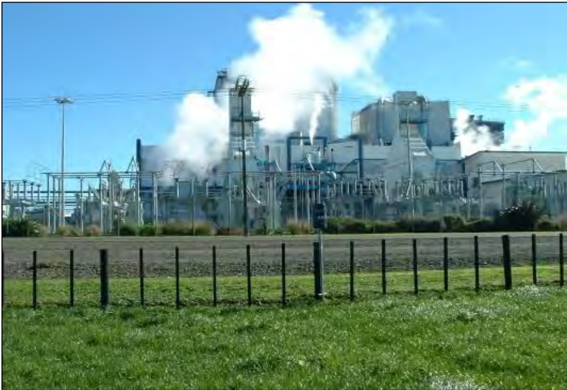
Photo 3 Air discharges from 'Cogen-I' and 'Cogen-II'
