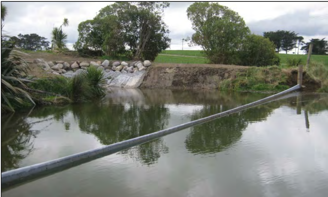
Photo 7 Tawhiti stormwater pond following remedial work
