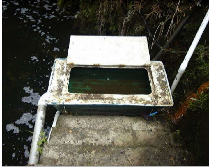
Photo 9 Elver trap at the base of the tail race at the power station
