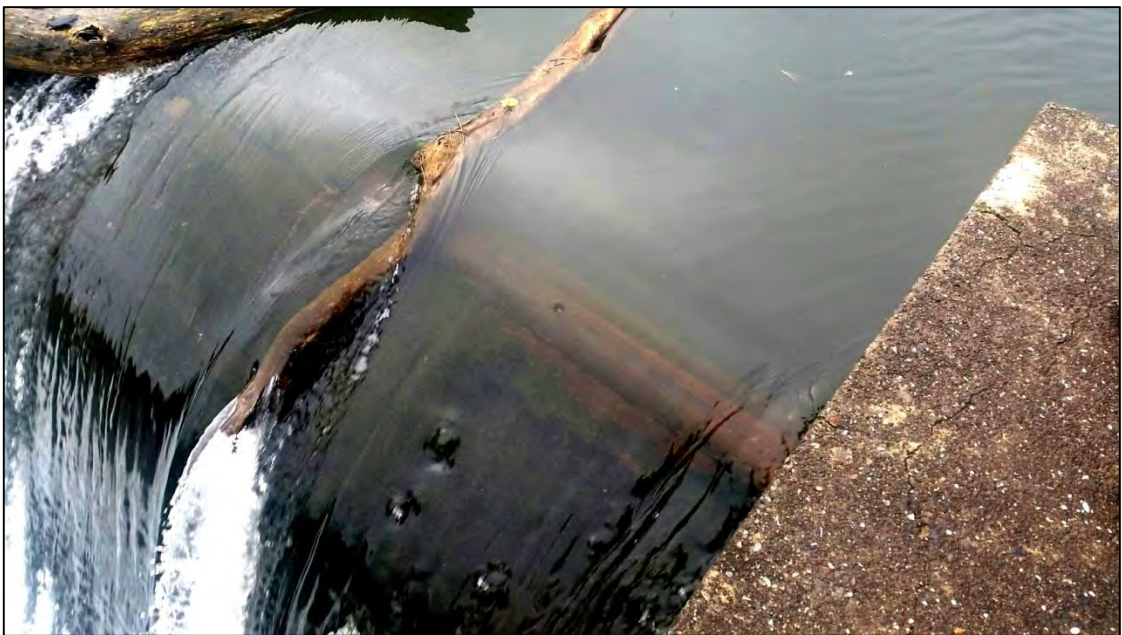
Photo 5 The baffle installed on the weir to improve lamprey passage
