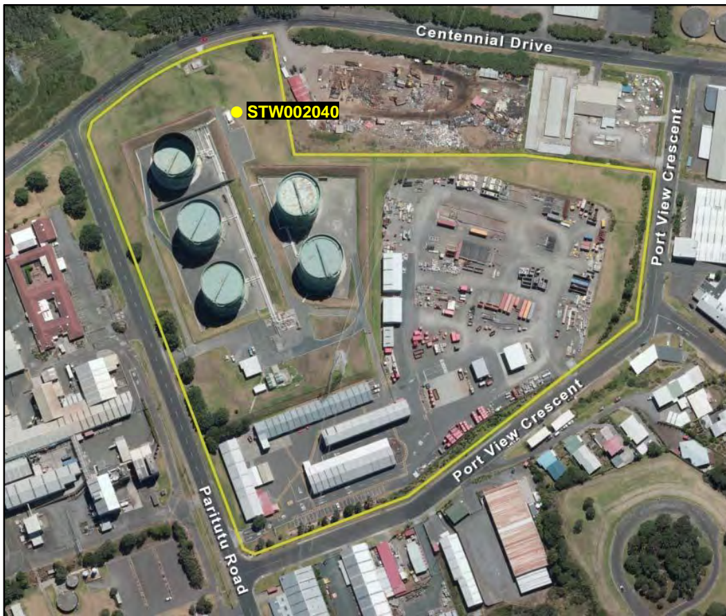
Figure 6 Aerial photograph of the Shell Todd Oil Services Ltd Paritutu Tank Farm
