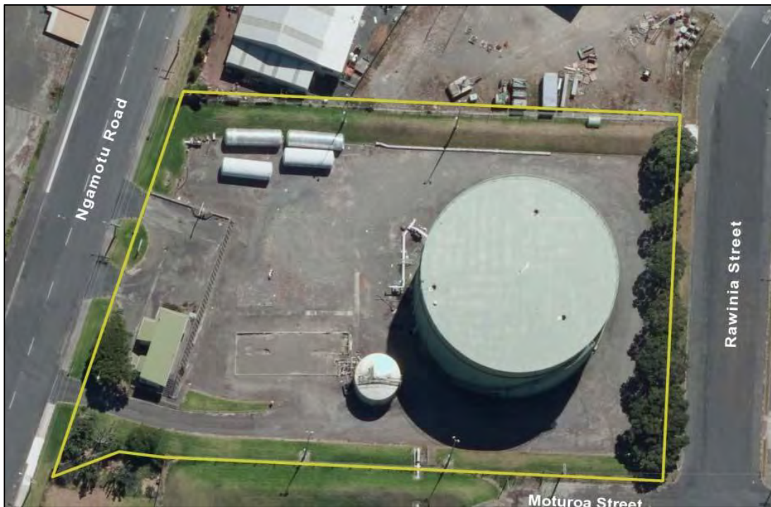
Figure 3 Aerial photograph of the Greymouth bulk storage facility
