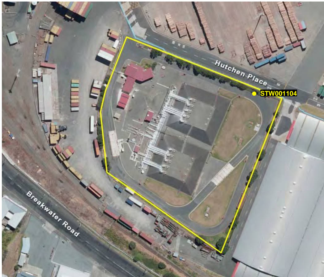
Figure 4 Liquigas site and sampling point
