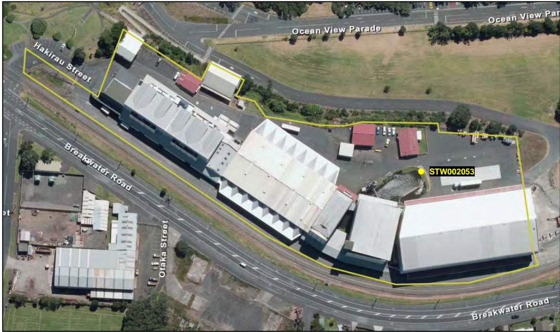
Figure 14 Aerial photograph of Fonterra New Plymouth Coolstores
