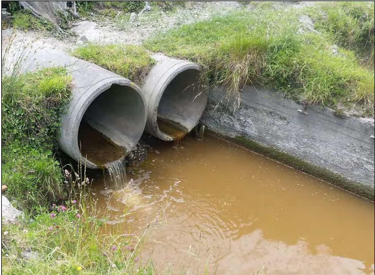
Photo 4 The access culvert immediately upstream of site 2, 9 December 2016.
