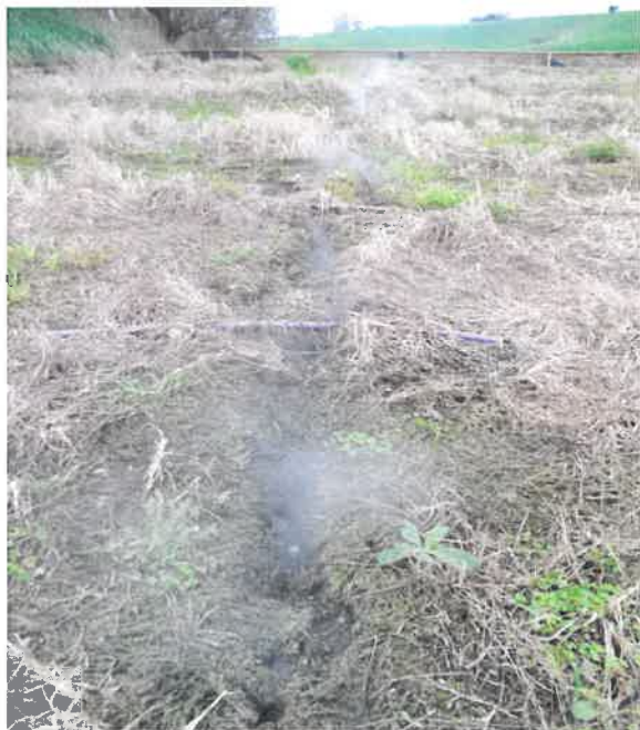
Figure 2: TBE concentrated. sources biofilter bed, with vapour leaking above one of the main ducts.
