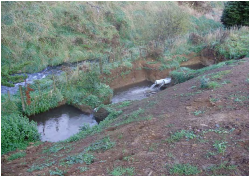
Photo 3 The settling system at Taranaki Fish and Game trout hatchery
