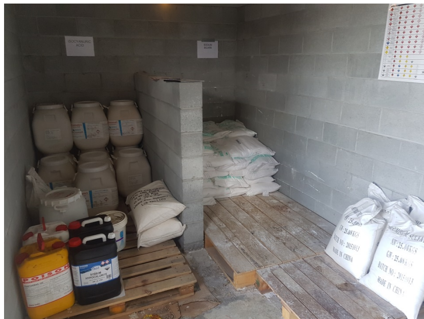
Photo 2 Inspection of chemical storage shed, 12 May 2016
