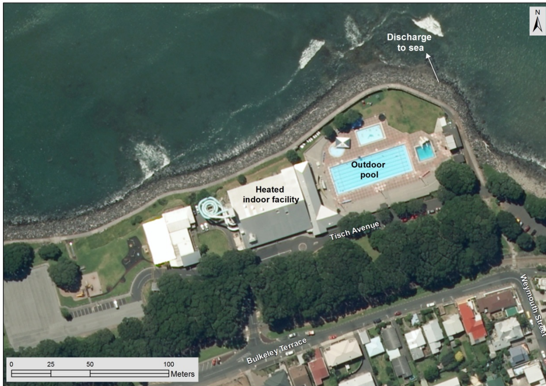
Figure 1 Location of Todd Energy Aquatic Centre
