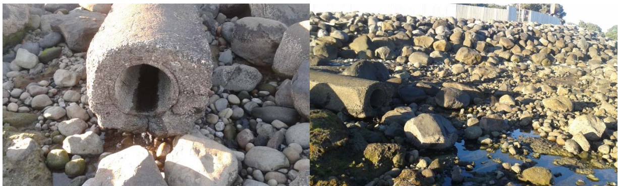
Photo 2 Discharge from marine outfall
