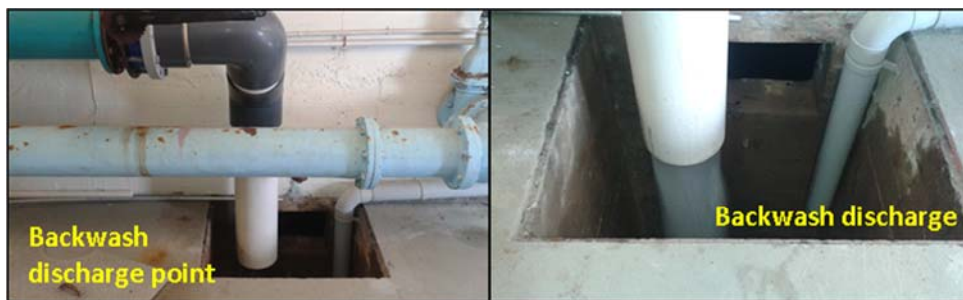
Photo 1 Discharge sampling point
