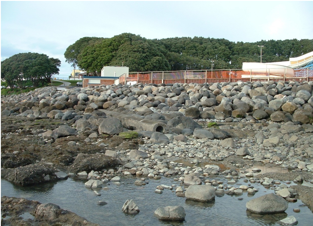
Photo 1 Todd Energy Aquatic Centre ocean outfall
