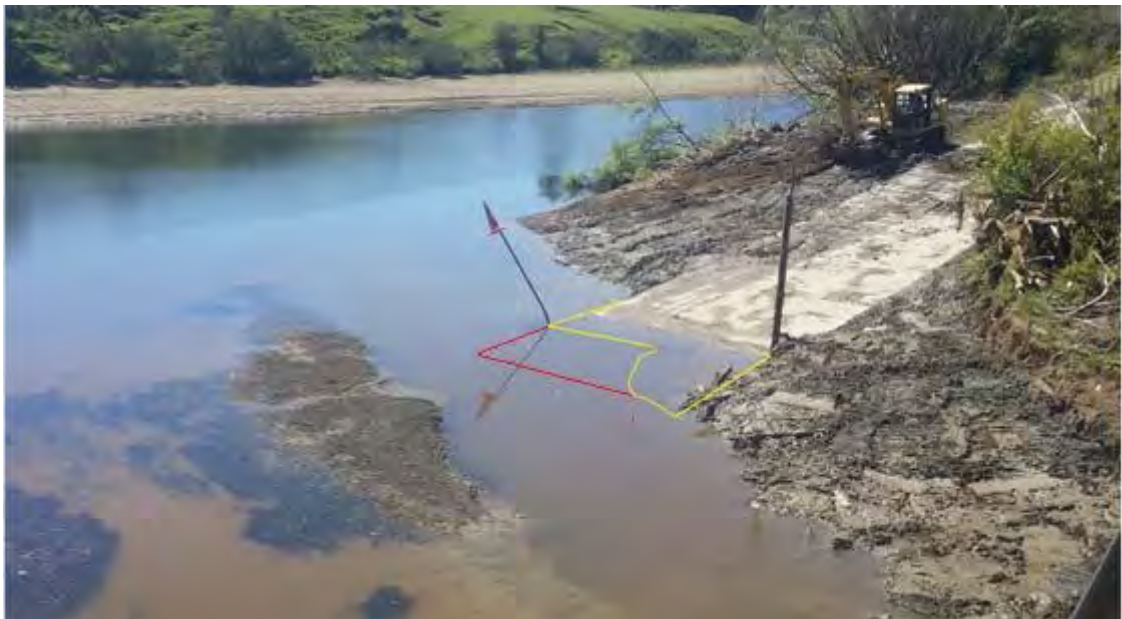
Photo 1 The Glen Nui boat ramp during a low lake level. The yellow line approximates the edge of the concrete ramp pre-improvements, the red line the edge of the ramp post-improvements.
