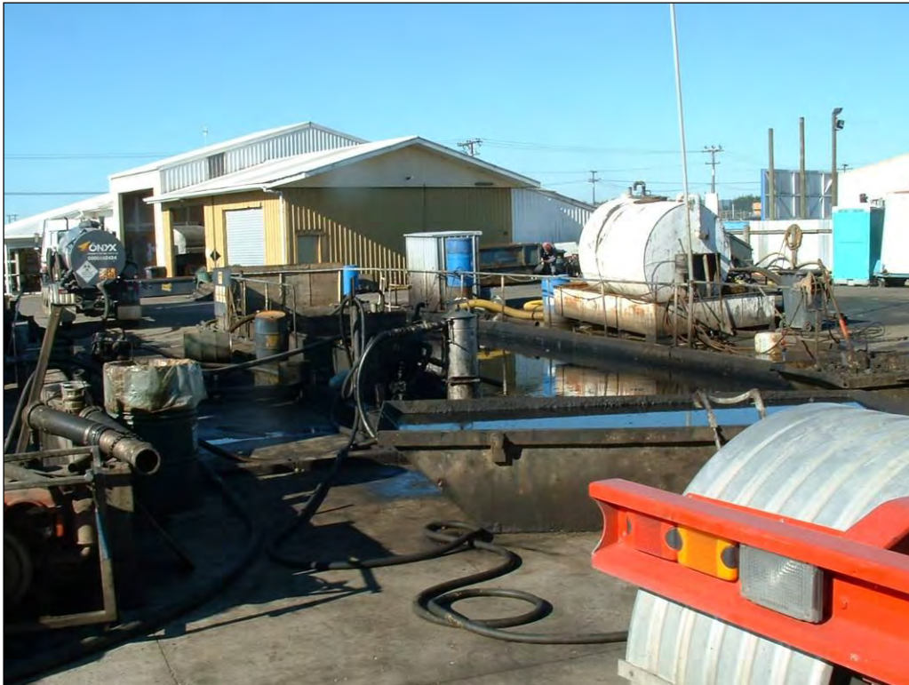
Photo 3 Intergroup Ltd oil treatment facility
