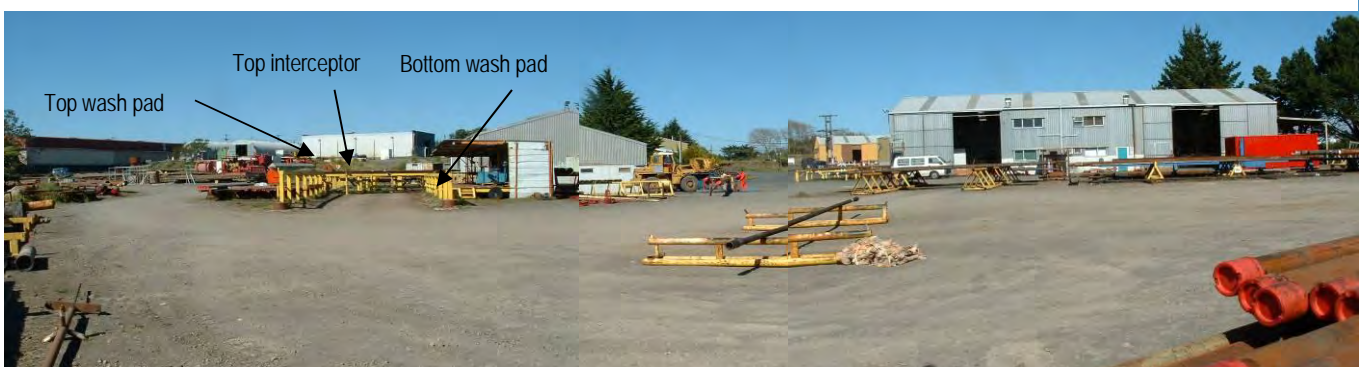
Photo 5 Weatherford - view from the northern corner
