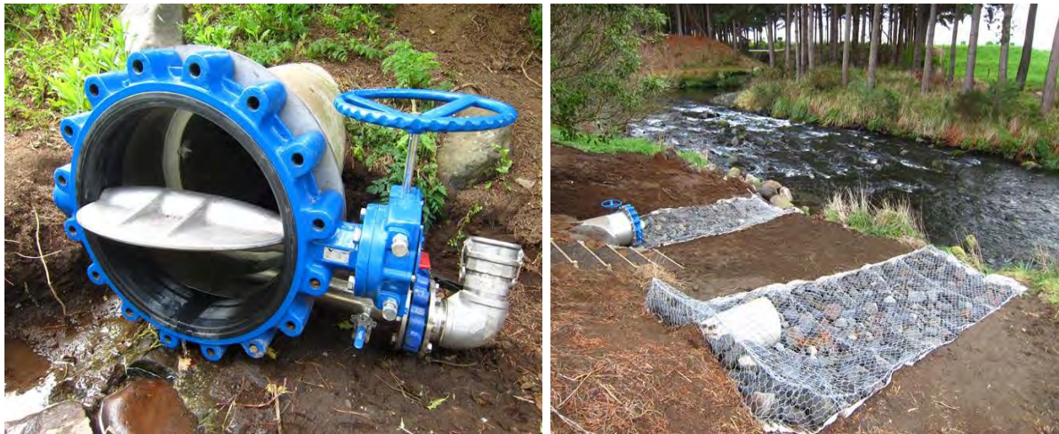
Photo 1 Valve on northern storm drain, and Reno mattresses laid out below storm drains to Kaupokonui Stream
