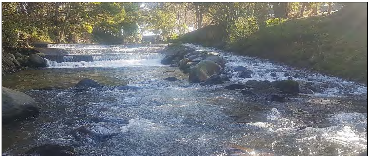
Figure 1 Kaupokonui Stream, Kapuni Lactose weir and fish pass
