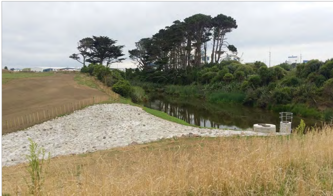
Photo 6 Southern stormwater pond following upgrade (surrounded by native riparian plantings)
