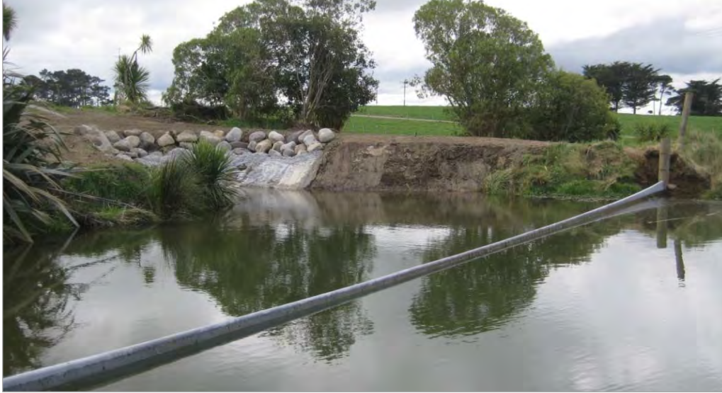
Photo 7 Tawhiti stormwater pond following remedial work
