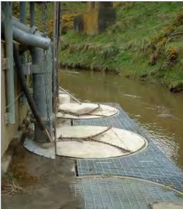
Photo 5 Tangahoe River intake
