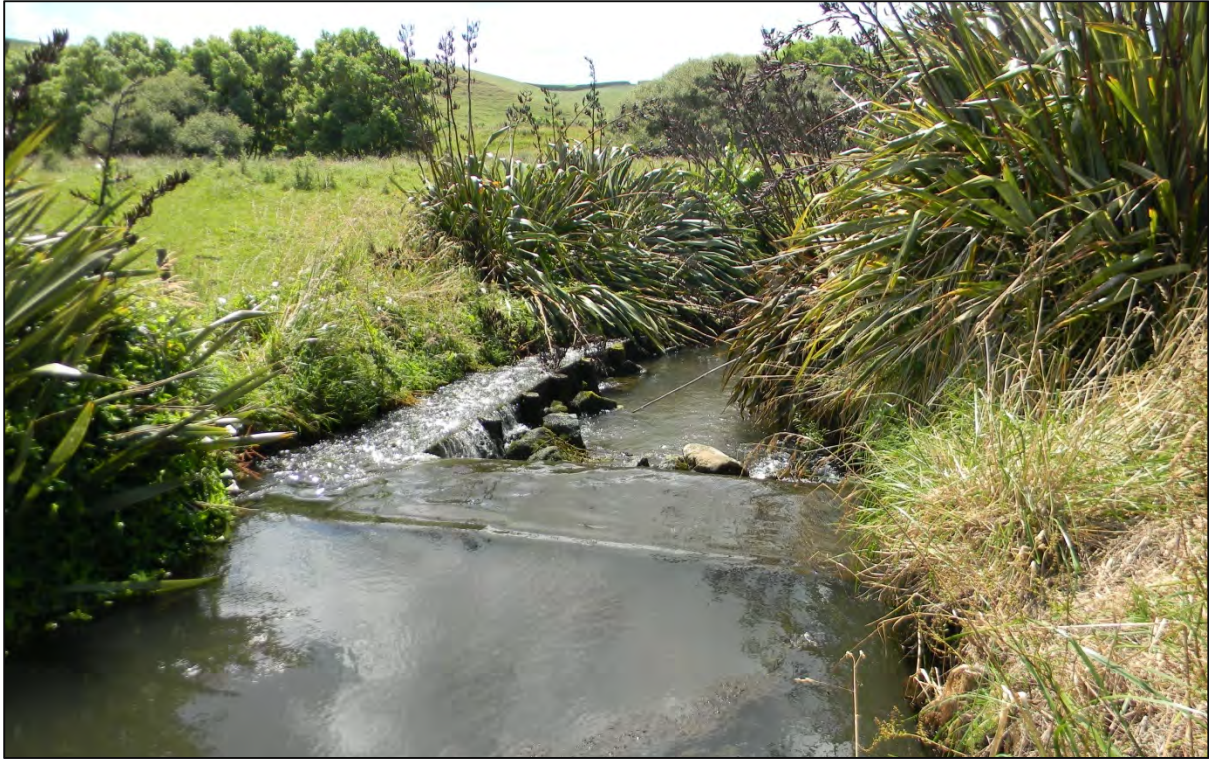
Photo 1 The weir and fish pass on the Tawhiti Stream
