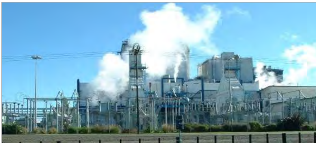
Photo 3 Air discharges from 'Cogen-I' and 'Cogen-II'
