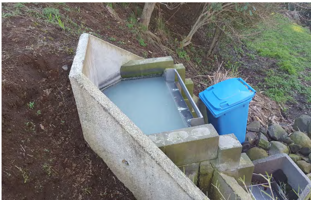
Photo 3 Turbid white discharge to wetland observed during inspection on 10 August 2016
