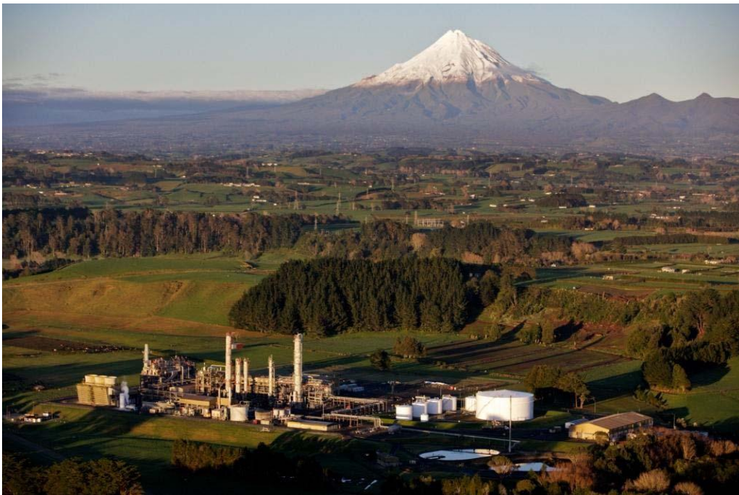
Photo 3 Methanex Waitara Valley site
