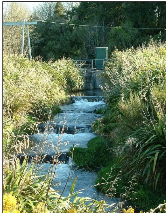
Photograph 1 The new fish pass (8 September 2010)
