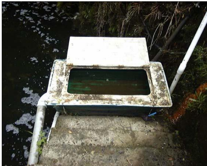
Photograph 3 Elver trap at the base of the tail race at the power station
