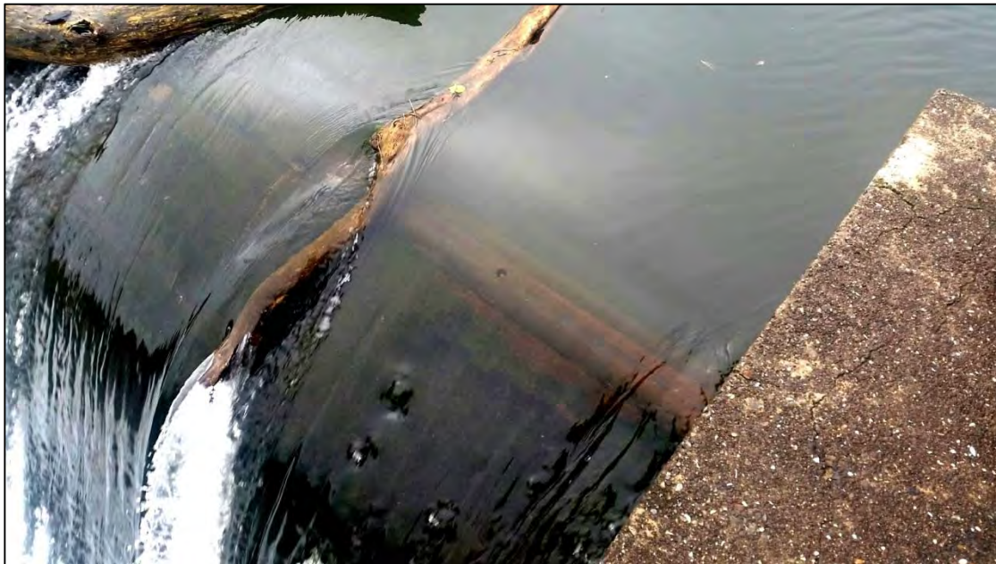
Photo 6 The baffle installed on the weir to improve lamprey passage
