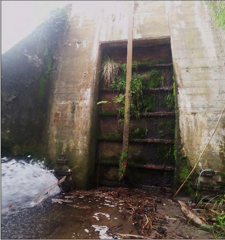
Photo 2 The sluice gate on the true left side of the weir, 21 September 2016
