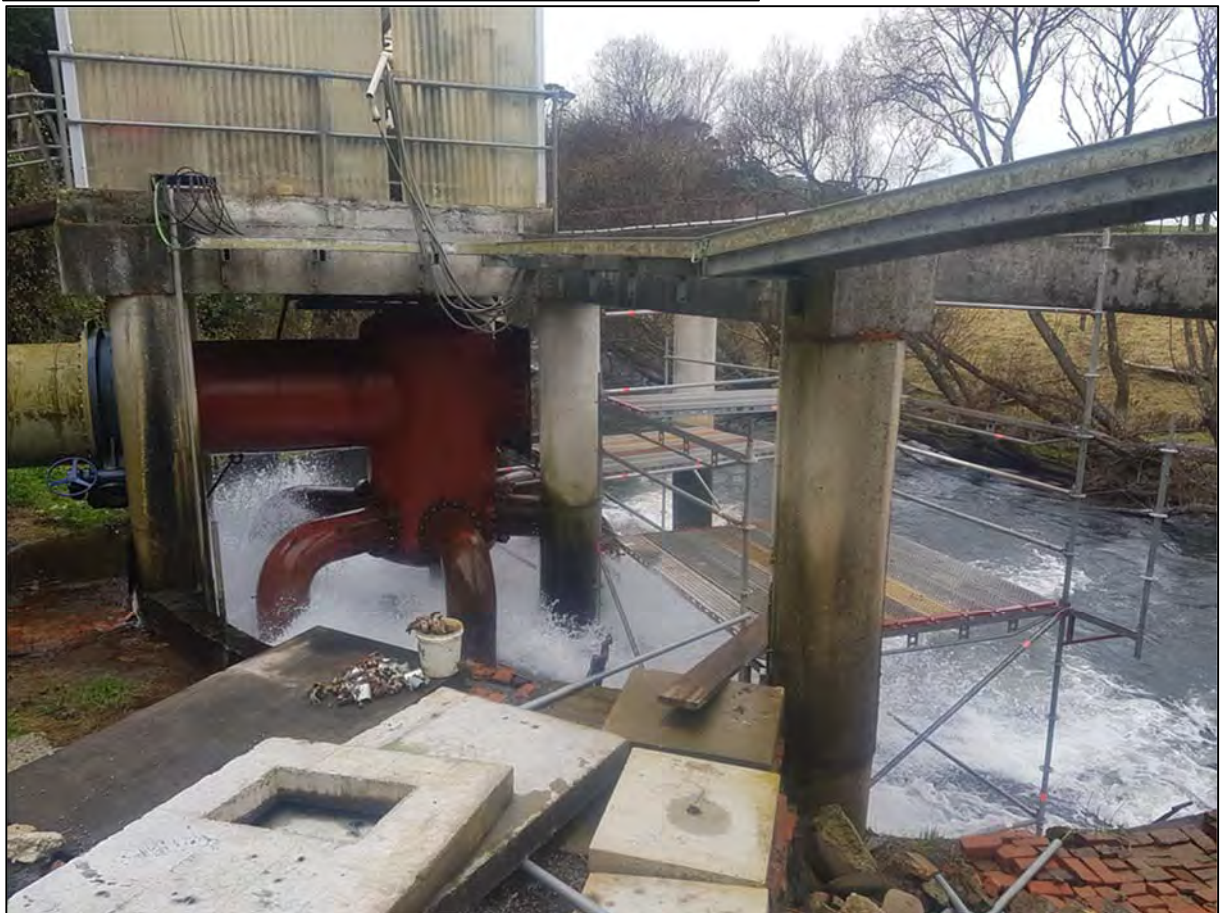
Photo 5 The station during the inspection of 12 May 2017
