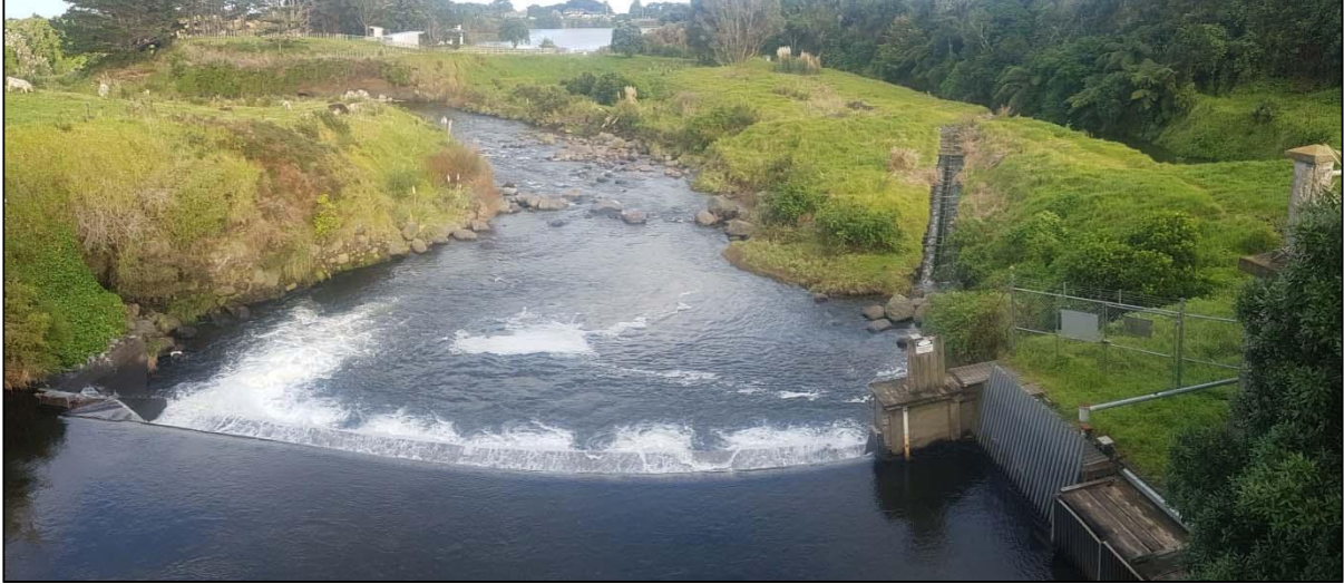
Photo 1 The Waiaua River, weir, intake, canal, fish pass and Lake Opunake, as viewed from the State Highway 45 Bridge, Opunake.
