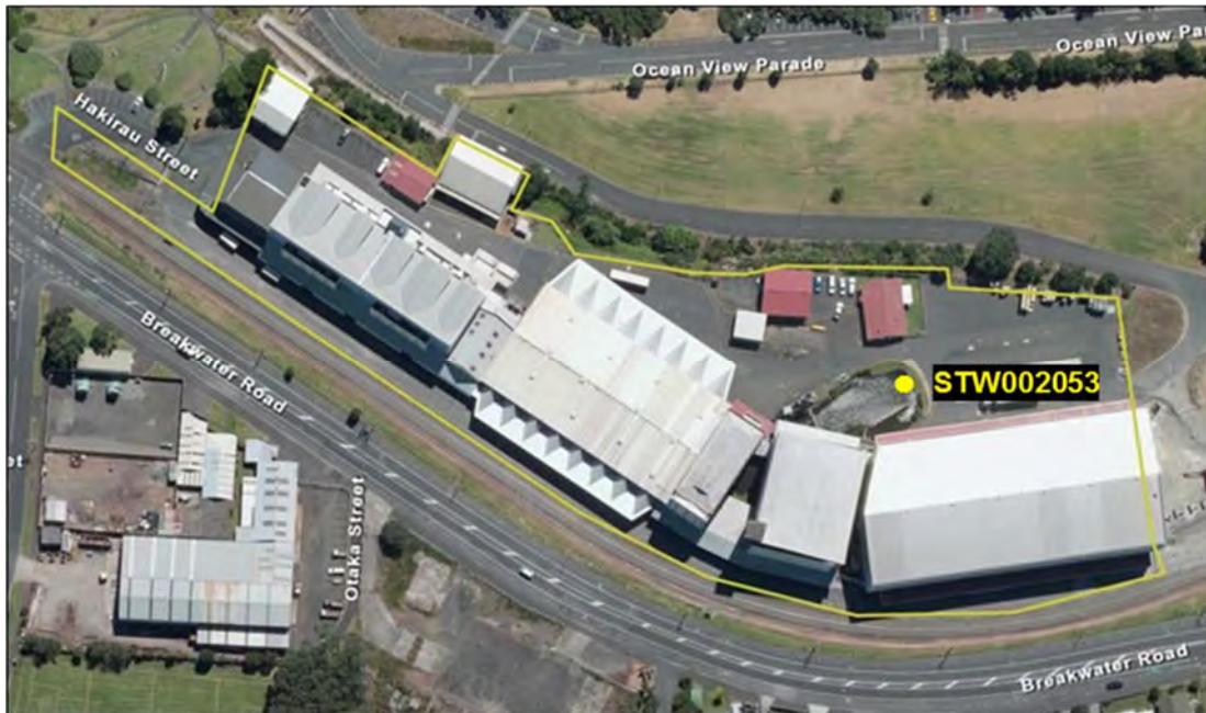
Figure 14 Aerial photograph of Fonterra New Plymouth Coolstores
