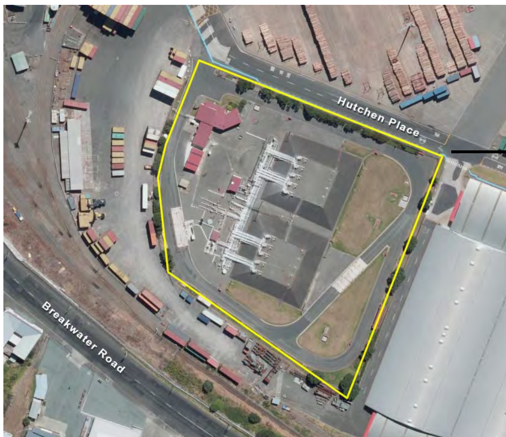
Figure 4 Liquigas site and sampling point
