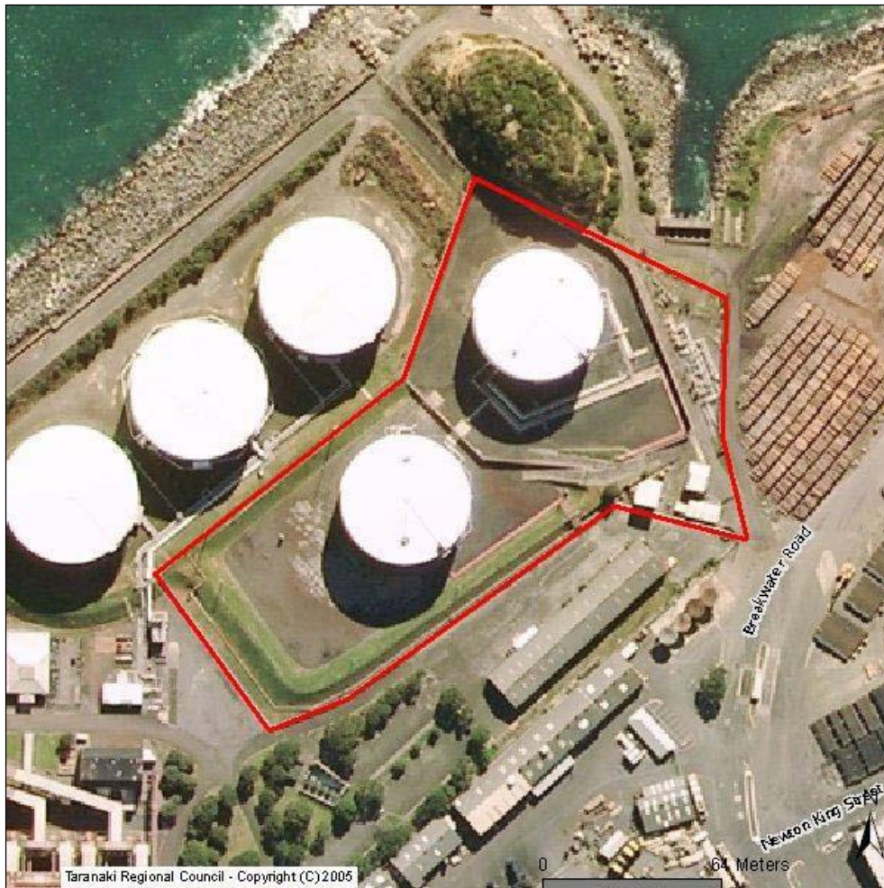
Figure 2 Aerial photograph of the Methanex New Zealand Ltd site at Port Taranaki
