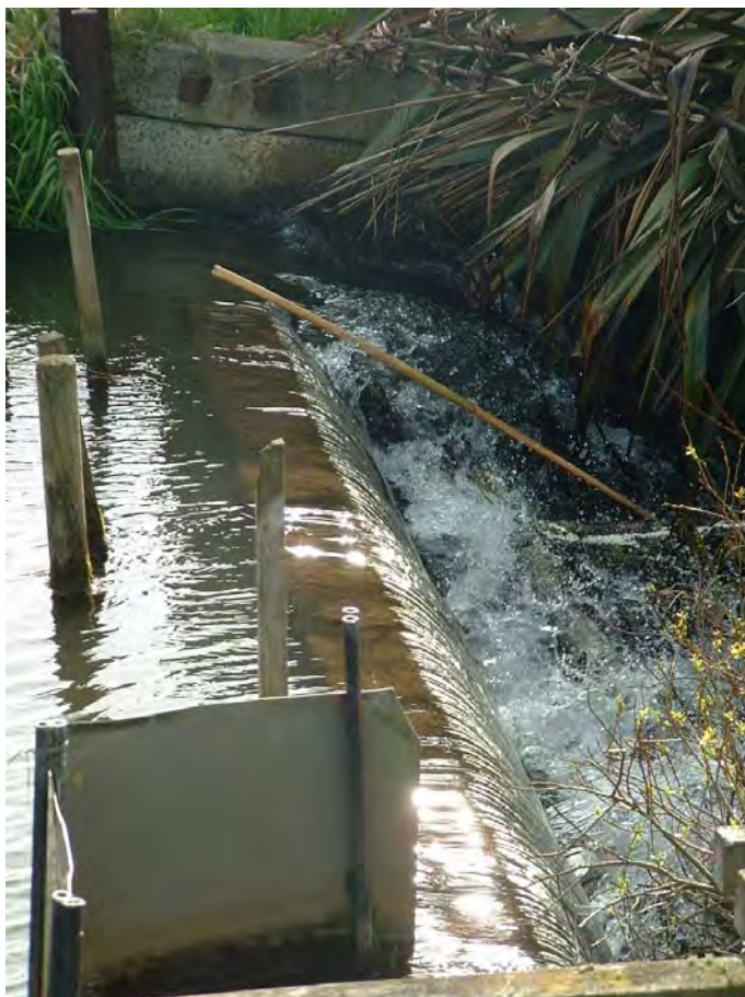
Photo 1 (left) The weir and fish pass on the Tawhiti Stream (fish pass visible on far side)
