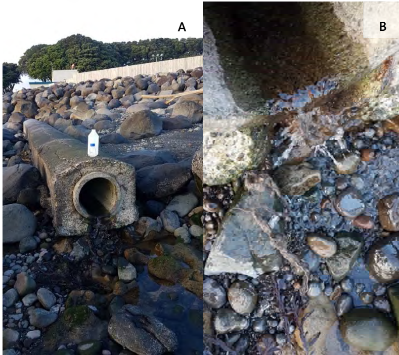
Photo 3 (A) Medium flow discharging from the outfall on 19 May 2017; (B) Close-up of water discharging from the outfall, with human hair visible in the vicinity of the outfall
