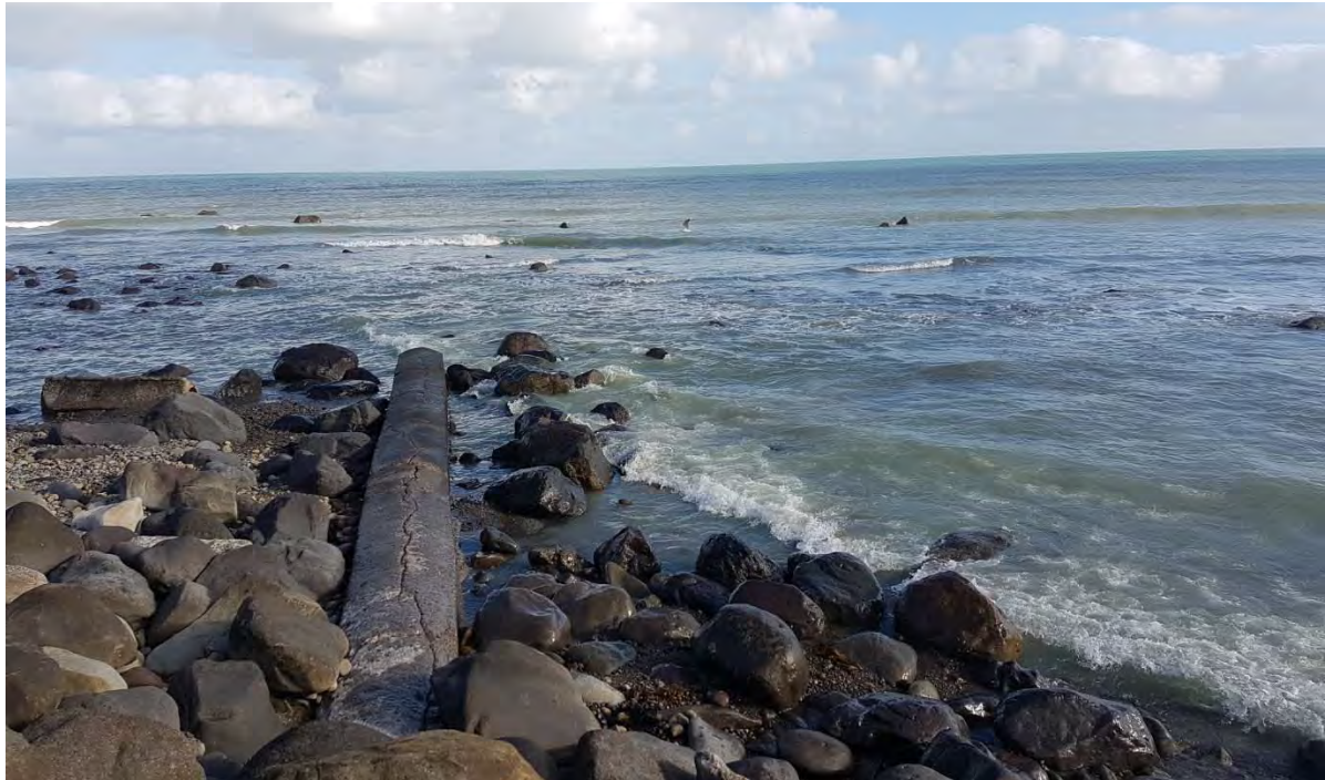
Photo 1 Outfall pipe at time of shoreline water sampling
