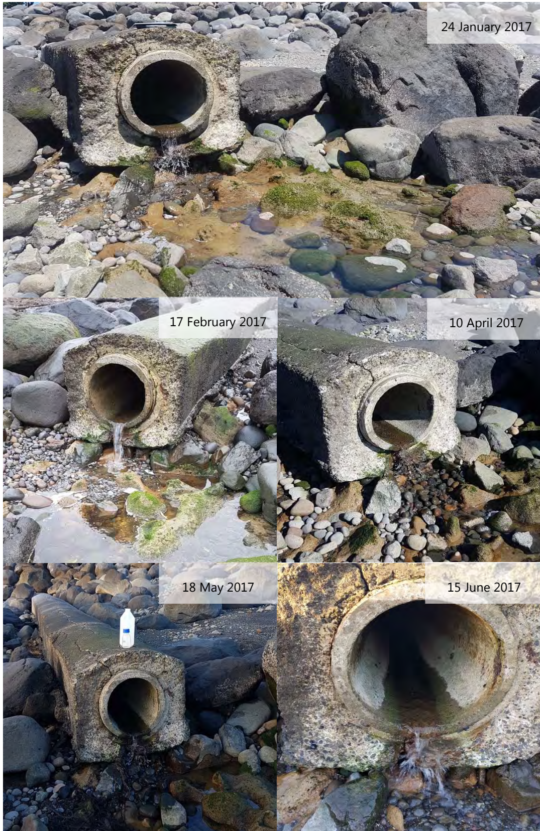
Figure 2 Water discharges observed occurring from the marine outfall pipe on the Kawaroa Reef during the 2016-2017 monitoring year
