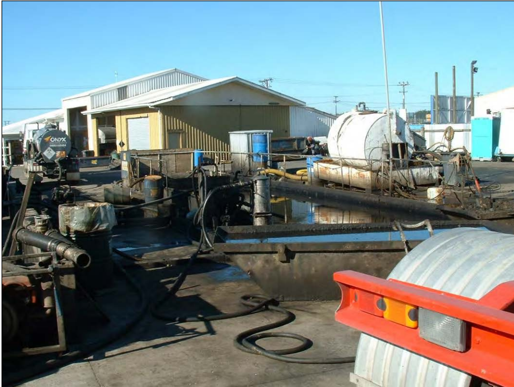
Photo 3 Intergroup Ltd oil treatment facility
