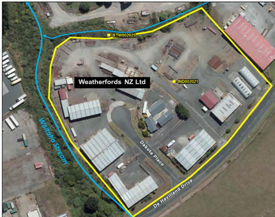
Figure 15 Aerial view of Weatherford's site
