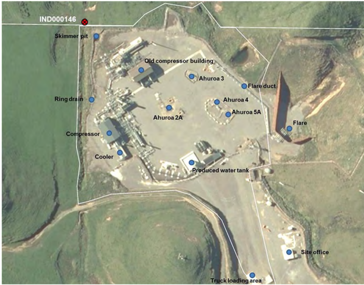
Figure 7 Ahuroa B wellsite and gas storage facilities
