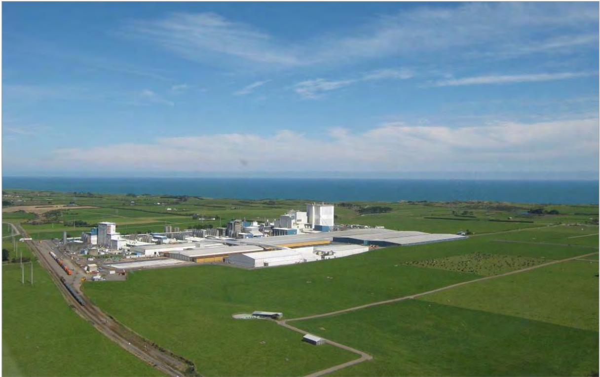
Photo 1 The Fonterra Whareroa site
