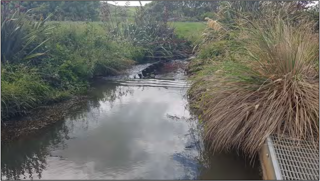
Photo 2 Tawhiti intake weir
