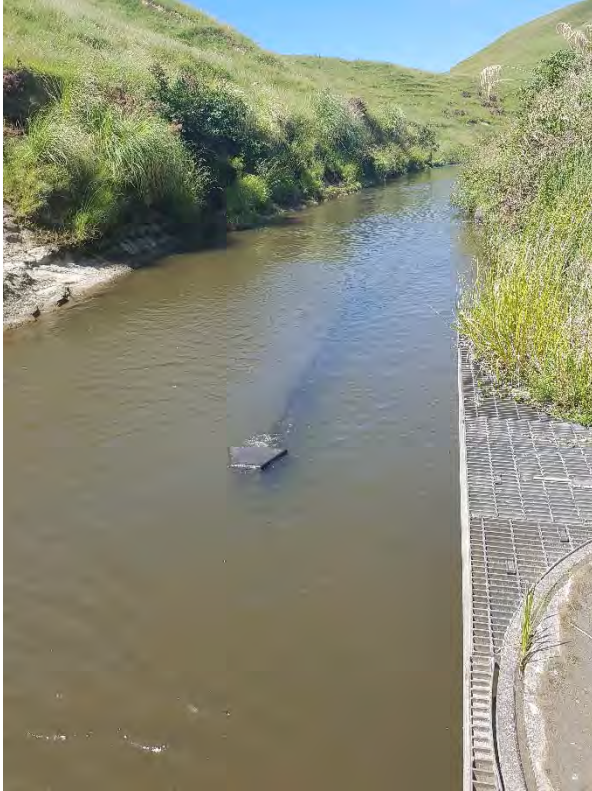
Photo 5 Tangahoe River intake
