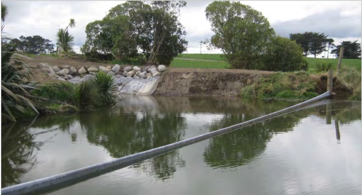
Photo 7 Tawhiti stormwater pond following remedial work
