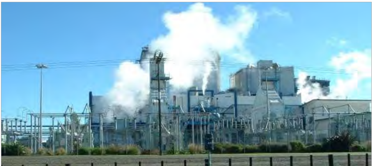
Photo 3 Air discharges from 'Cogen-I' and 'Cogen-II'
