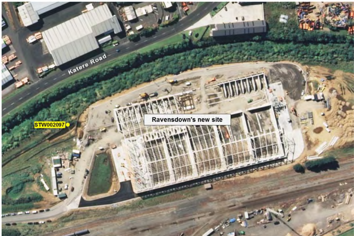
Figure 19 Ravensdown's new site location and discharge point
