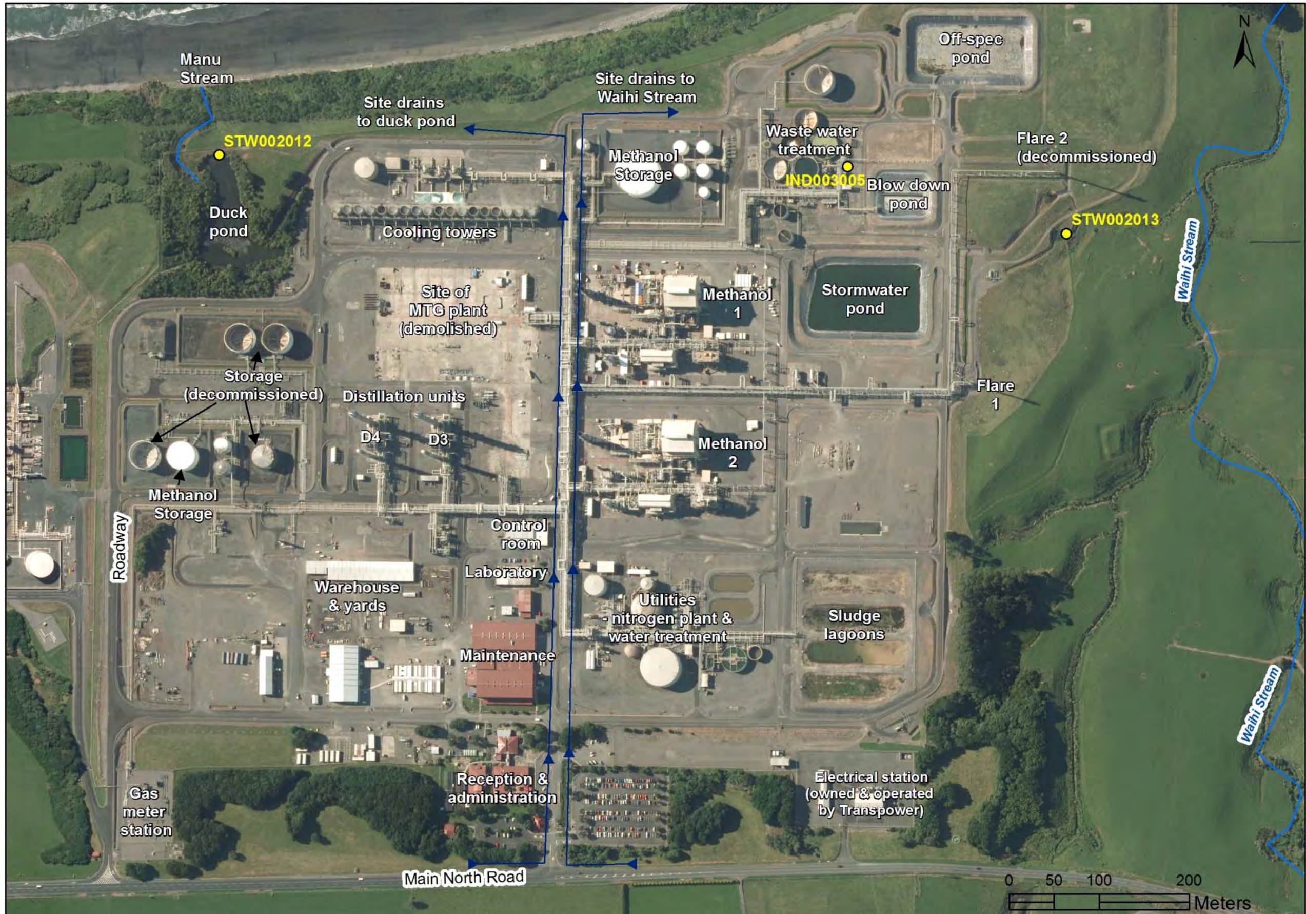
Figure 1 Motunui site layout and water sampling site locations
