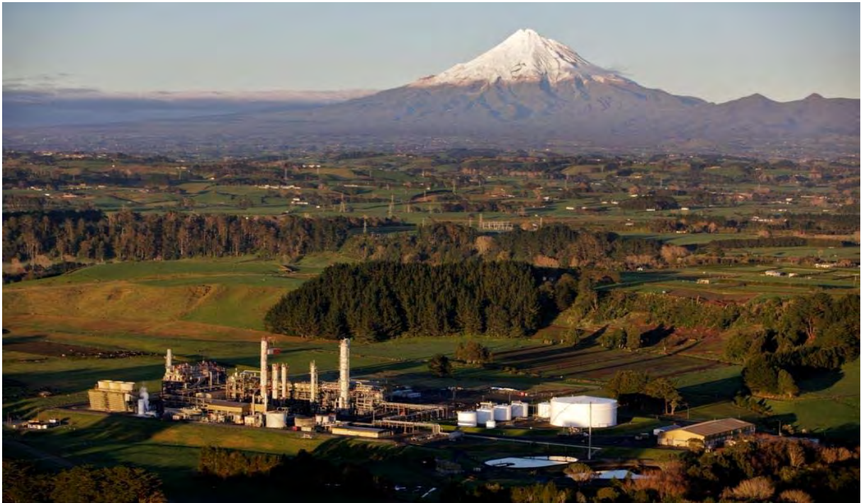
Photo 3 Methanex Waitara Valley site
